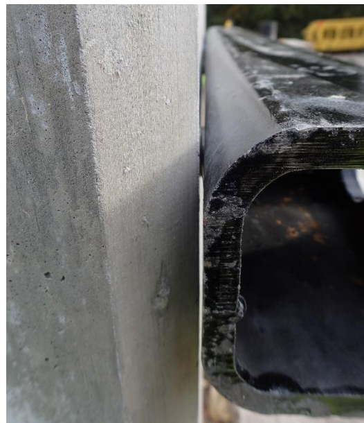
Figure 5.22: Waling beam mounting arrangement on face of trial panel.
