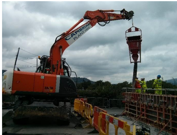
Figure 5.16: Reaction wall concrete pour.
