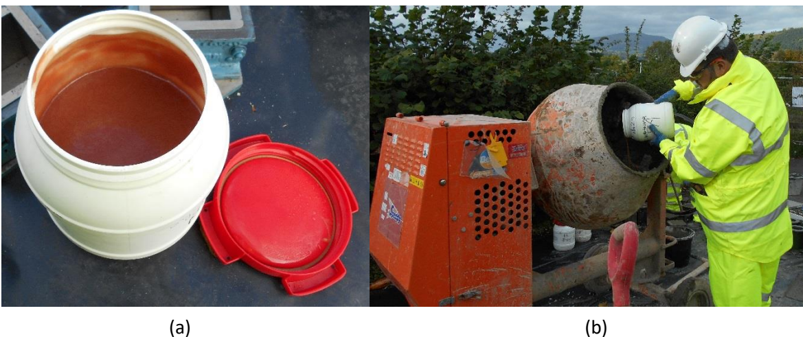
Figure 5.6: (a) Microcapsules in dispersion prior to mixing and (b) addition of microcapsules into the mix.
