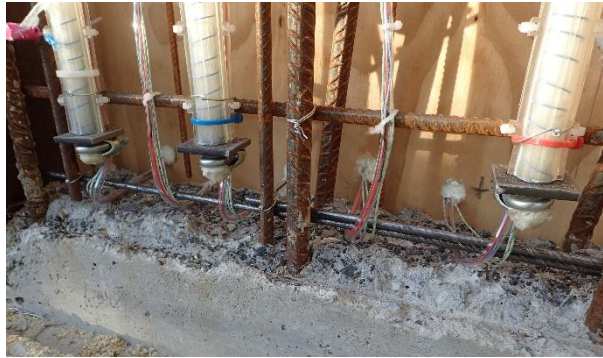
Figure 5.9: Set-up of polymer activation wires within formwork.
