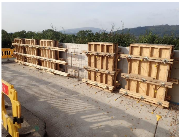
Figure 5.18: Trial panel formwork prior to concrete pour.
