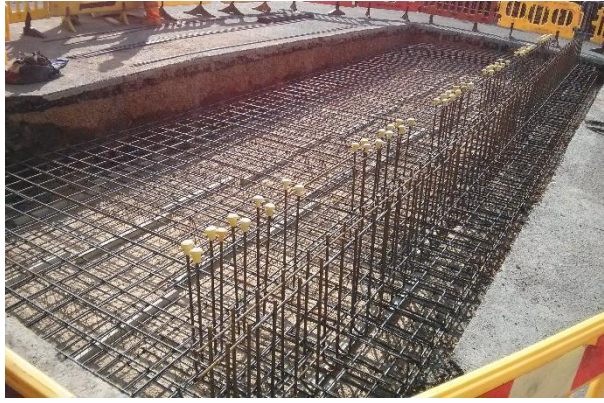
Figure 5.13: Base slab reinforcement.
