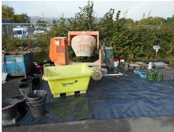
Figure 5.19: On-site concrete mixing set-up.
