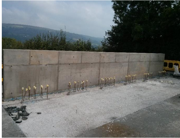
Figure 5.17: Reaction wall and base slab.
