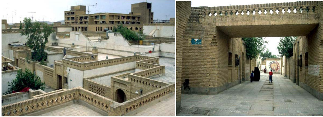
Fig. 3.36: Images of Shushtar New Town with narrow streets and roof level view of houses (source: AKDN 1986)
