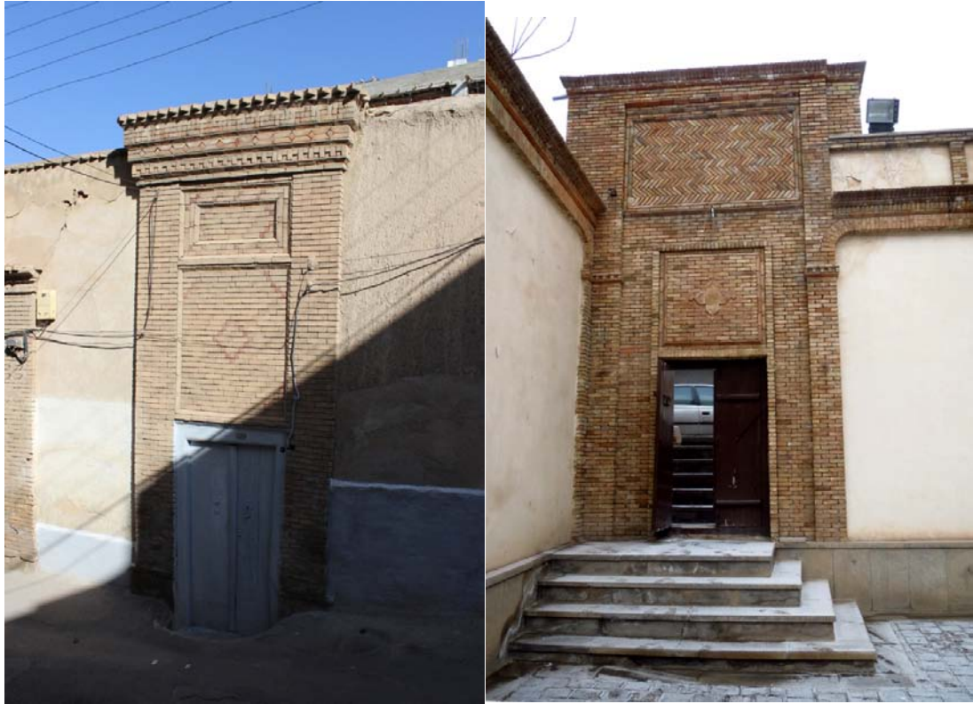
Fig. 3.5: A sunken front door from alleyway on left and stepped entrance to the courtyard on right from two houses in Tabriz (source: Author 2013)
