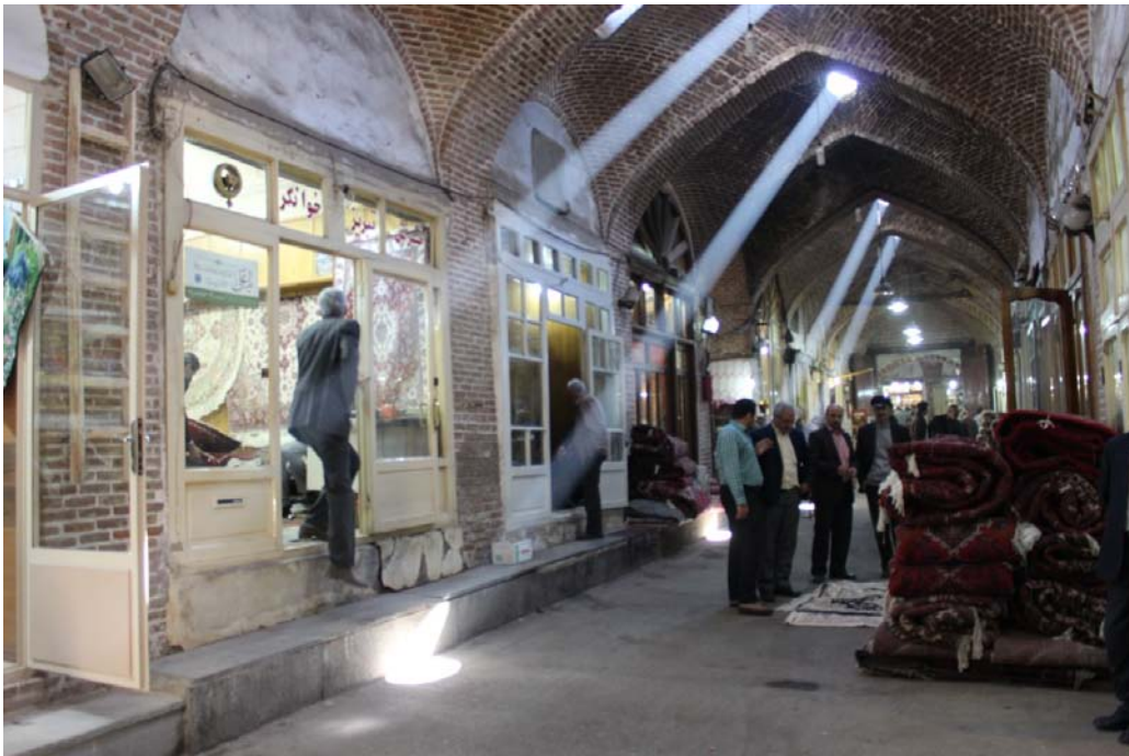
Fig. 3.11: Raste Bazaar covered with brick domes, Tabriz, Iran (source: Author 2013)
