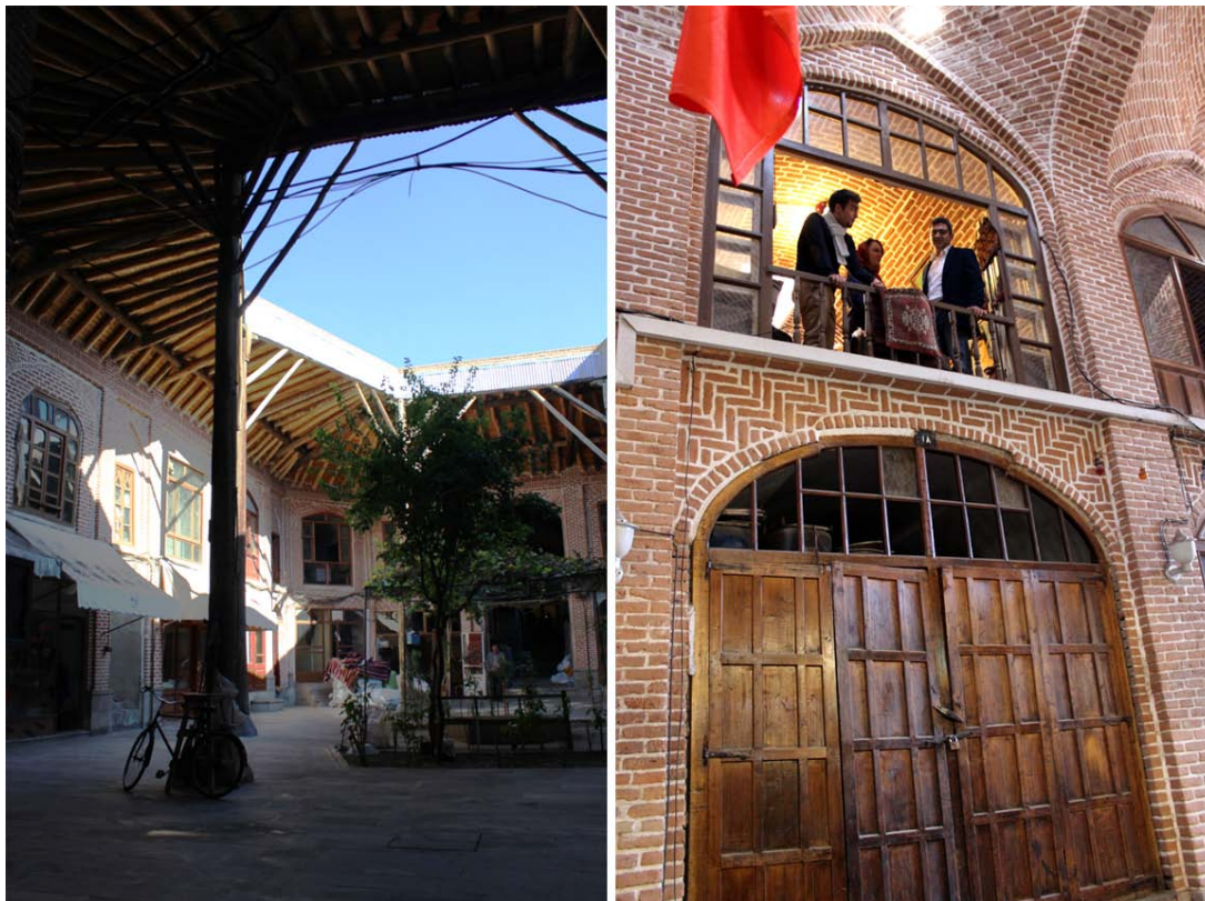
Fig. 2.29: Timber used in public buildings for posts, roof structure, doors and windows. Tabriz, Iran (source: Author 2013)
