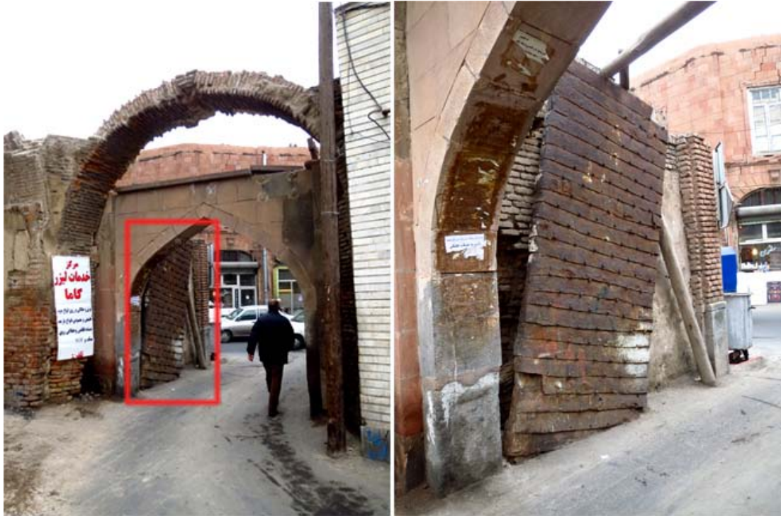
Fig. 3.1b: Part of historic city wall and Baghmishe gate in Tabriz seen at its current condition. The historic gate is a metal-clad timber gate which is currently buried under road surface (source: Author 2015)
