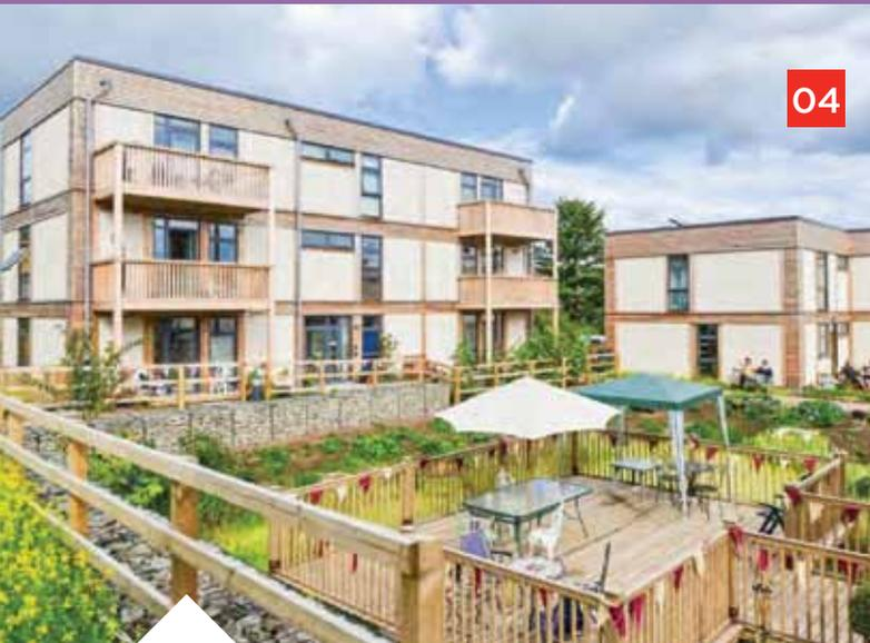
The completed LILAC project, made from straw-based panels assembled at a flying factory nearby, with rainwater harvesting and SUDs at its heart. [www.lilac.coop](http://www.lilac.coop)
