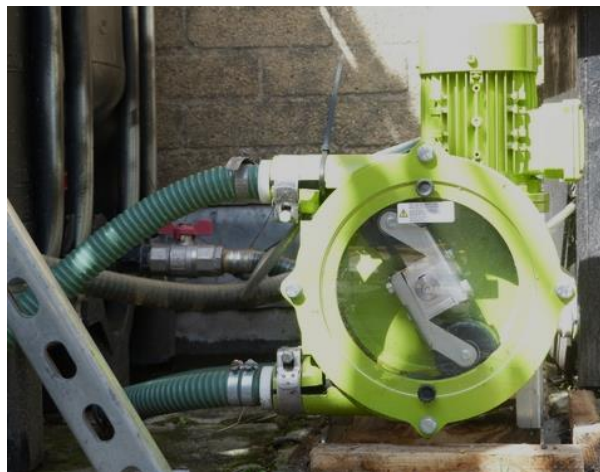
Figure 3.8 Peristaltic loading pump at University system
