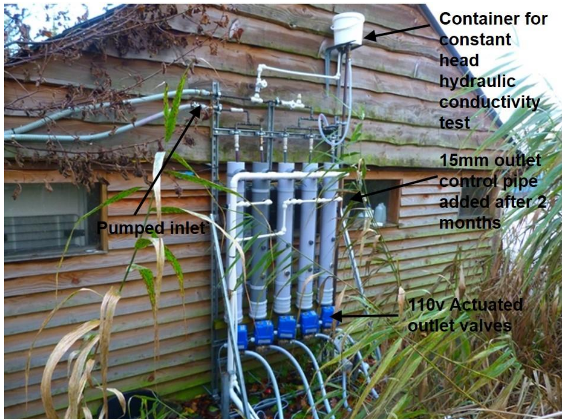
Figure 3.4 Model columns installed at site near Abergavenny
