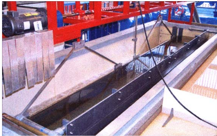
(b) Weir gate in operation
