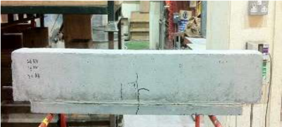
Figure 7.16 Beam sustained 1000000 cycles with some cracks (maximum cyclic load level 60.99%)
