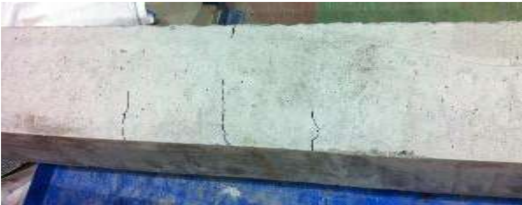
Figure 7.5 Beam sustained 1000000 cycles with some minor cracks
