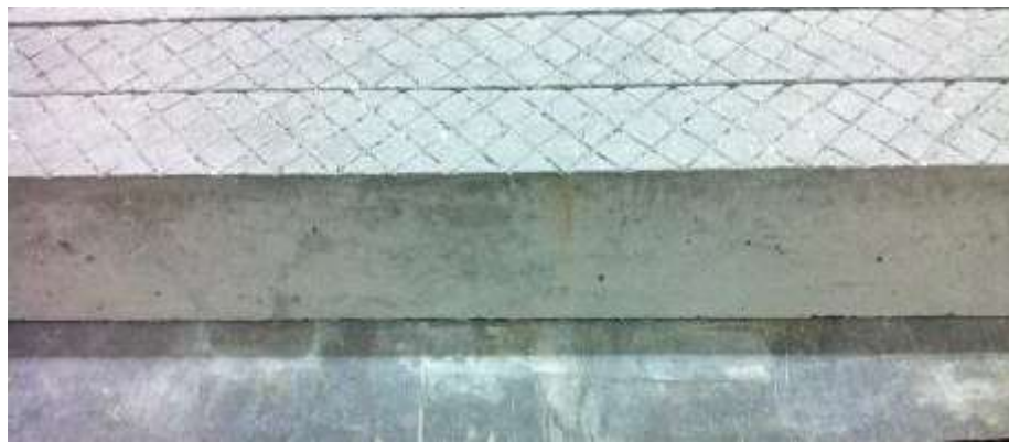
Figure 7.12 A grid of diagonal grooves to roughen the surface for bonding
