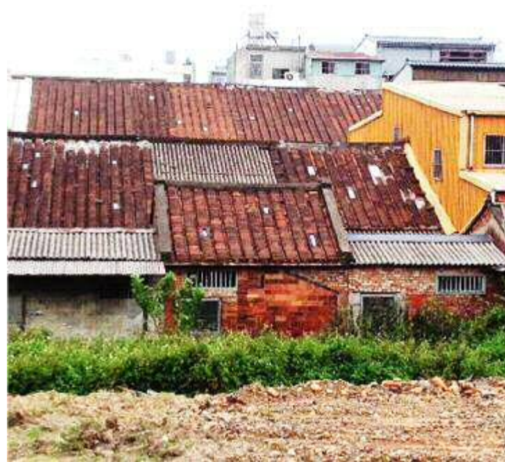
(b) Southern back-view of shophouses
