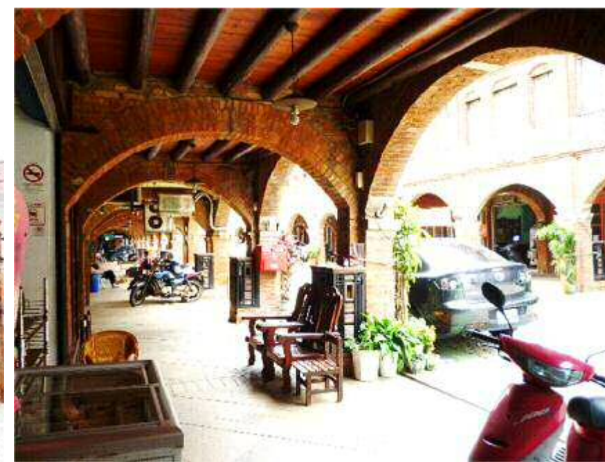
(d) View of covered walkways
