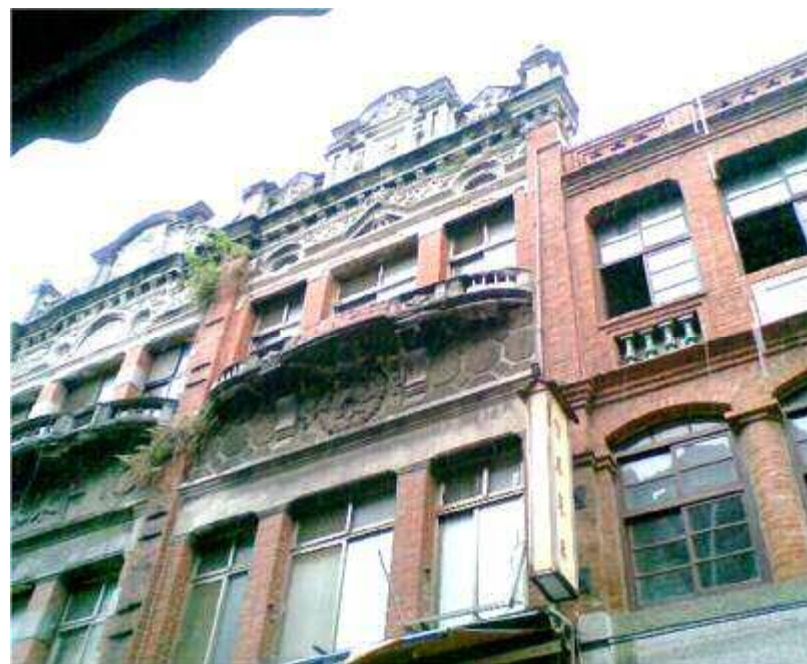
(b) Typical façade of shophouses
