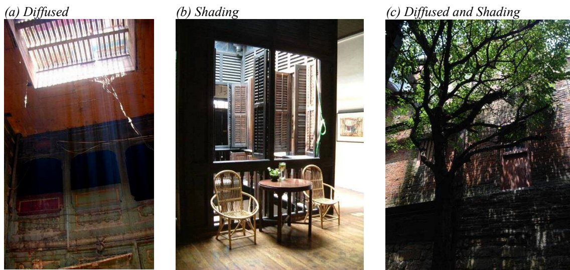
Figure 9.26: A well-designed shading system can reduce glare and generate dramatic interplay of light: (a) diffused light through horizontal louvers in a poor temple, Georgetown of Penang; (b) sun shading by wooden shutters blinds, the Cheng Hoe Seah Heritage building, Penang; and (c) sun shading by tree, the Bo Pi Liao historic district, Taipei City, Taiwan. (Source: Photographs taken by author, 2008-12)
