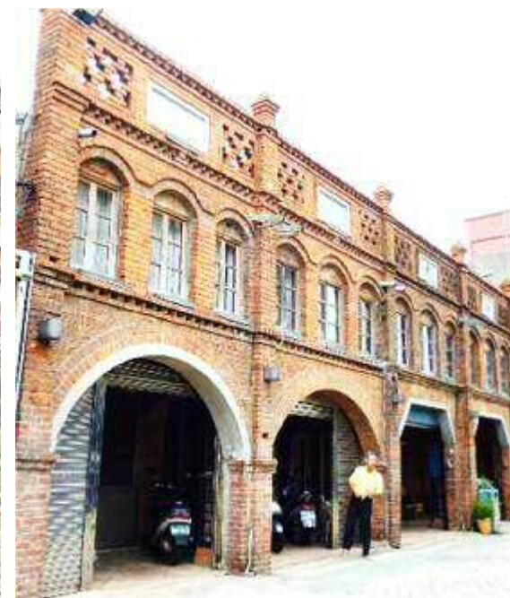
(c) Street view at east end
