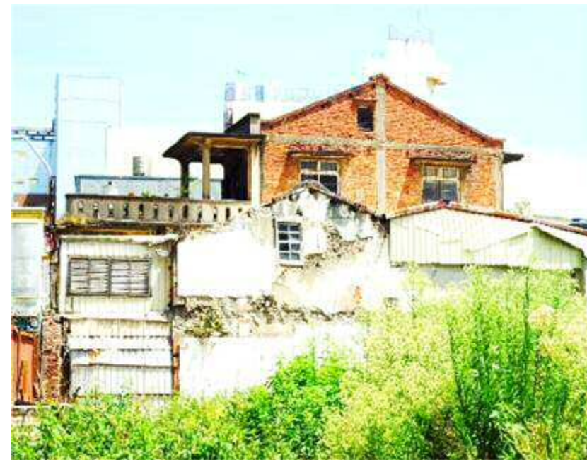
(d) No. 144 and 146, were partly destroyed
