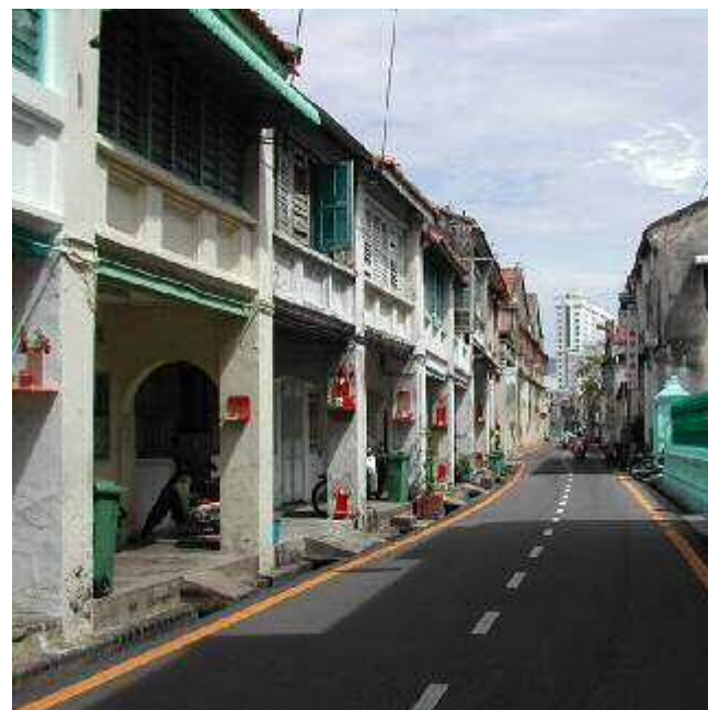
(b) Streetscape of residential buildings
