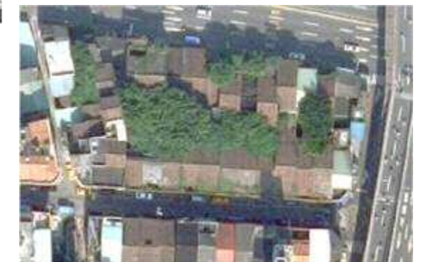
(e) Original and typical block of shophouse
