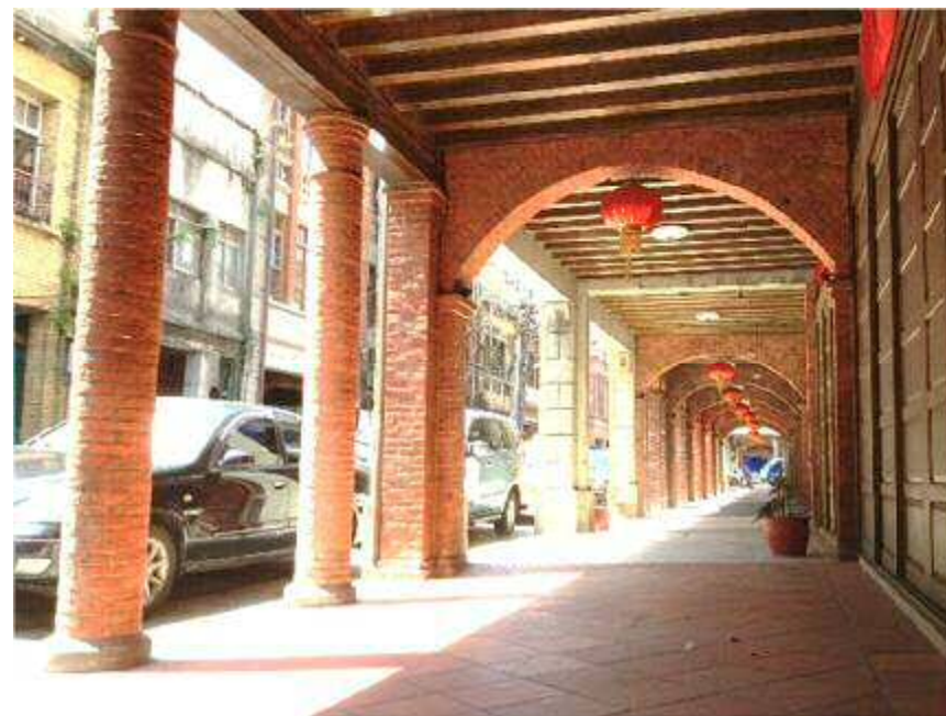
(c) Renovated walkways at northern end of the street
