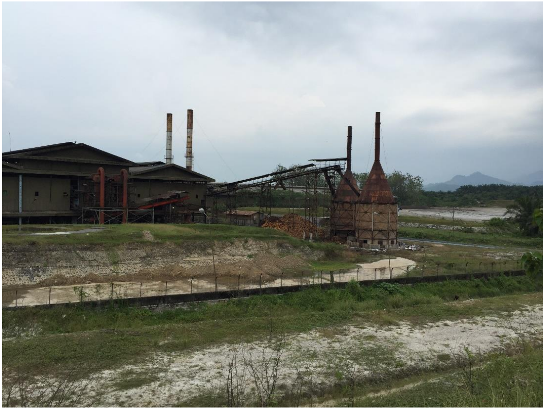
Image 5.1: A palm oil refinery in North Sumatra, Indonesia
