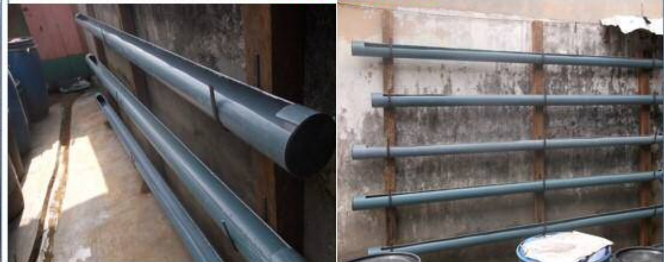
8: Images on Site 3
