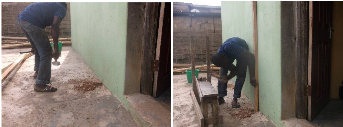
Plate 6-7; Digging foundation and placing 'hardwood barriers', source, Author, 2014
