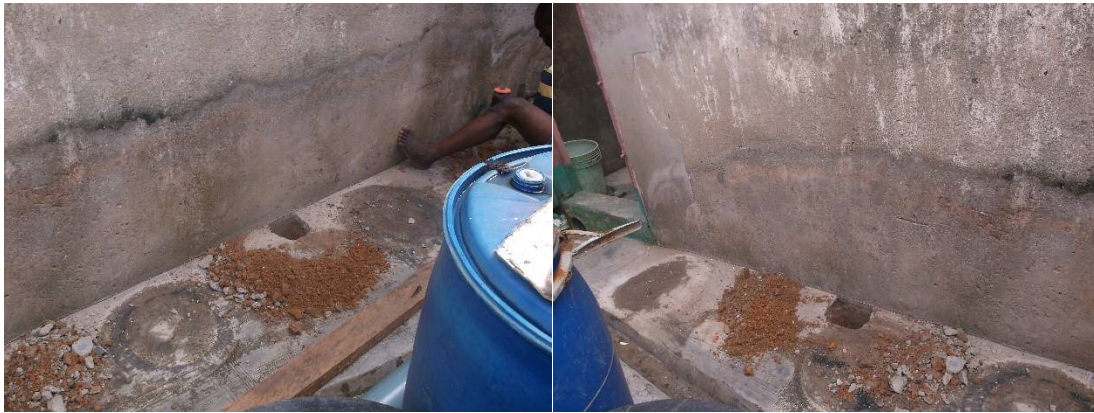
Plate 6-6; Holes dug for mini foundation, source, Author, 2014
