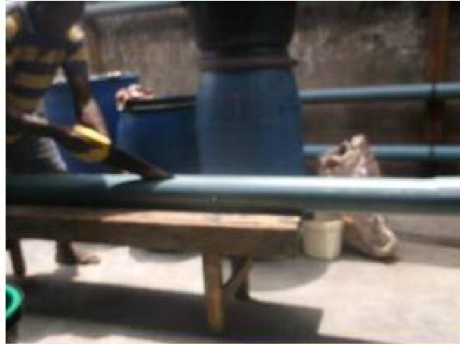
Cutting open the HDPE pipes with the use of Saw
