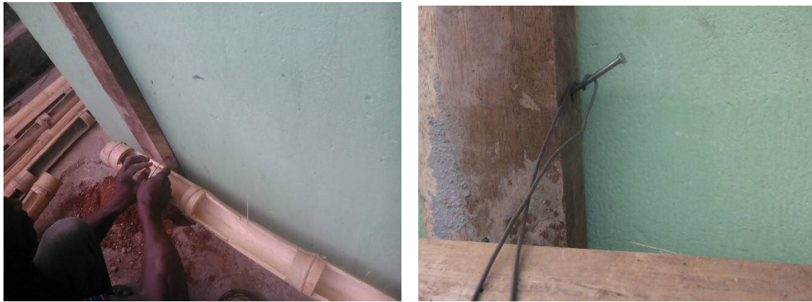
Plate 6-11; Anchoring binding wires to hardwood support, source: Author, 2014
