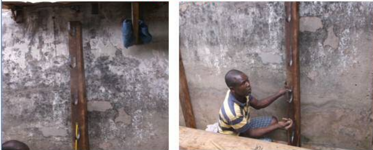
7: Images on Site 2
