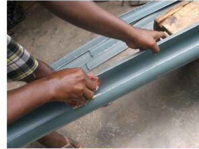
Clearing debris from HDPE pipe
