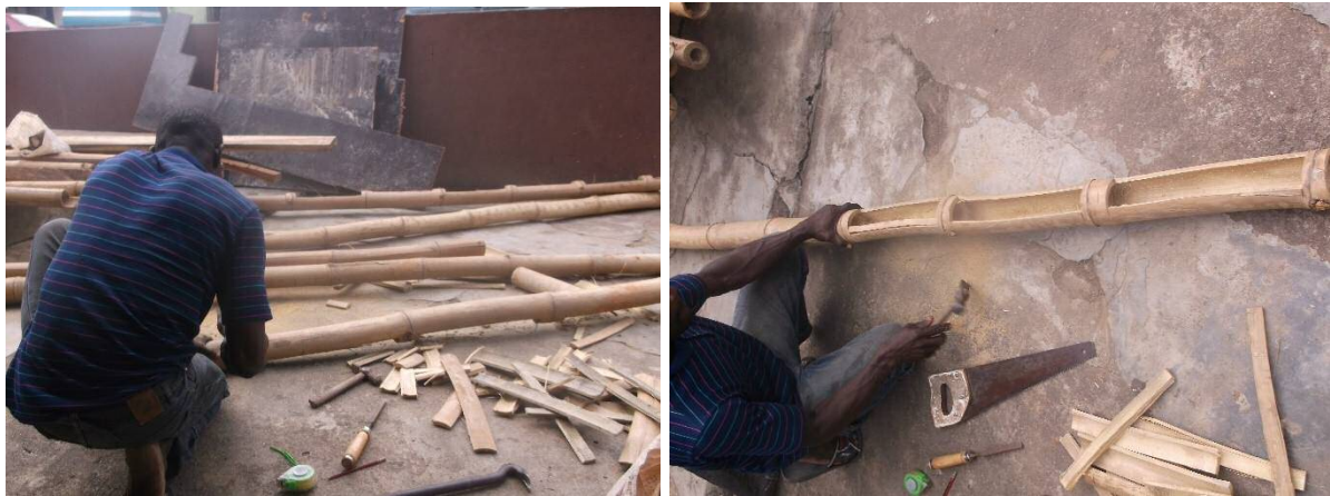
Plate 6-9; Marking Bamboo wood and cutting along joints, source: Author, 2014
