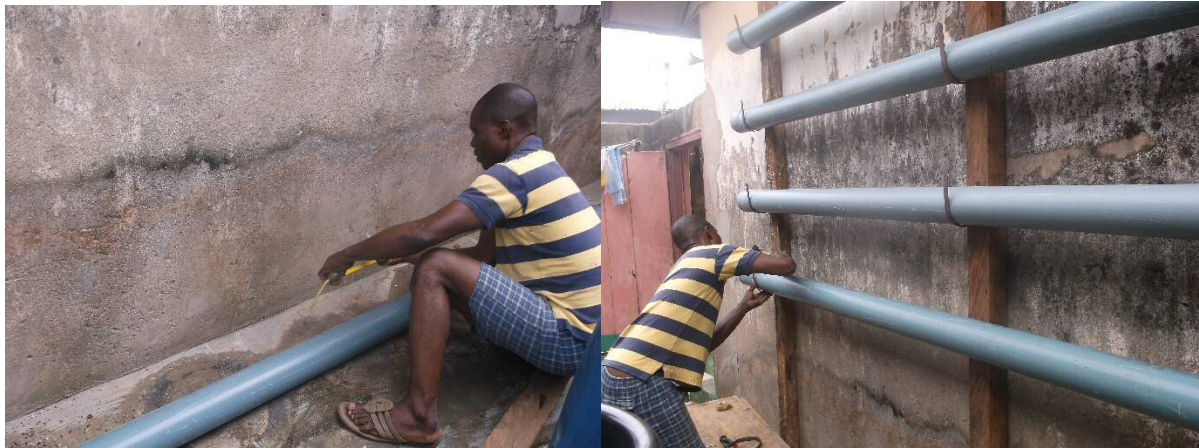
Plate 6-8: Marking HDPE pipes for area to be cut out, source: Author, 2014
