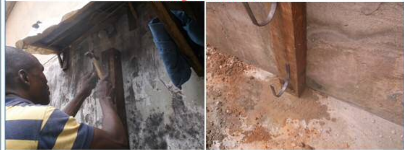
6: Images on Site 1
