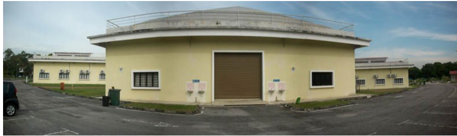
Figure 4.50 Studio 3 Industrial Design Building
