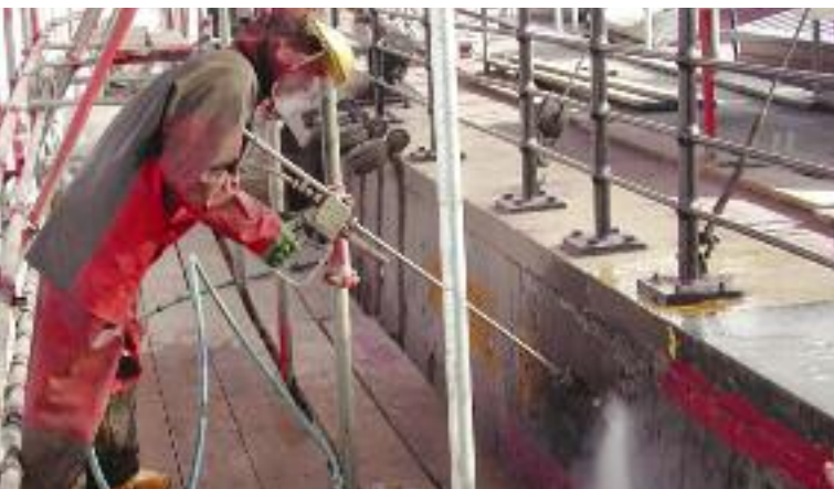
Figure 9. Preparing the upper hull for painting (image courtesy of Eura Conservation)
