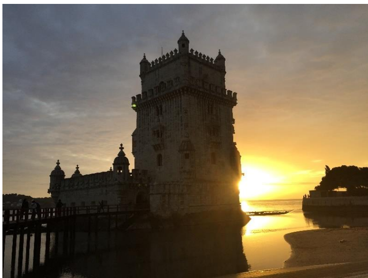
Figure 23: overview of Belème tower in Lisbon
