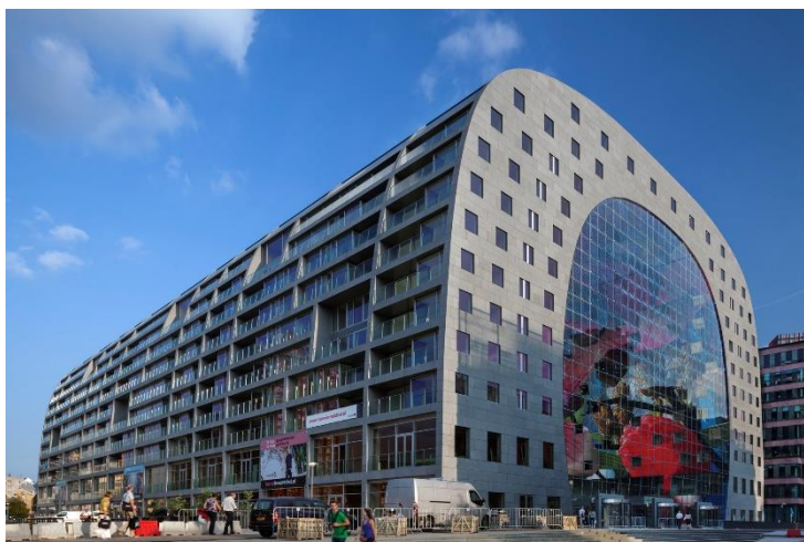
Figure 18 the Rotterdam market hall
