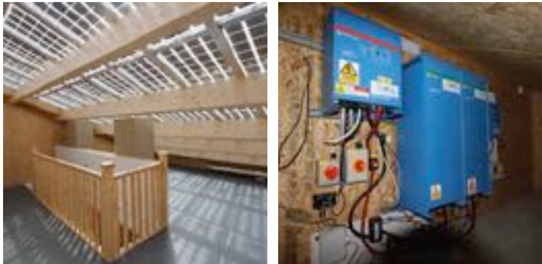
Figure 112 – Photos of the glazed mono-crystalline PV and LFP battery systems installed in the Solcer House.
