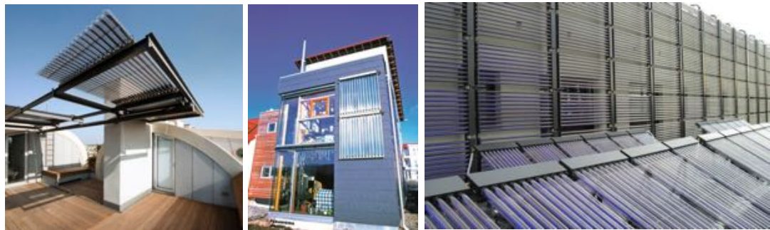
Figure 46 – Refrigerant-based BIST collectors: Heat pipe solar collectors integrated into the building as shading systems or double-skin facades.
