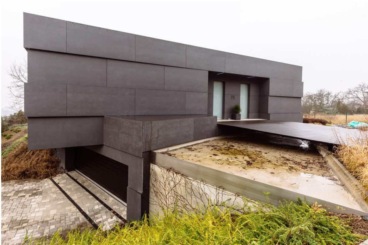
Figure 5: The Northern façade, its relation to ground and inhabitation of pool by algae (photo: Birke 2018)
