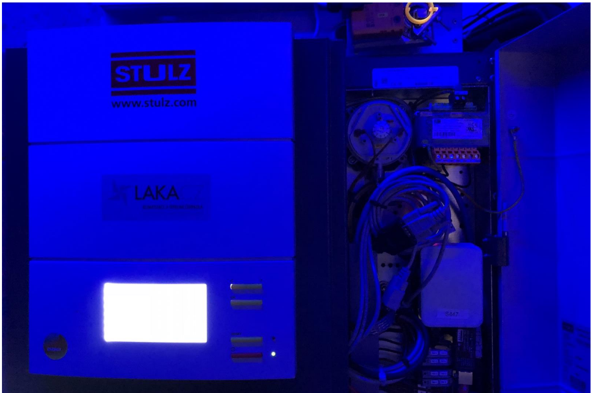
Figure 6: Prototype integration with datacenter precision A/C compartment using Modbus. (photo: Pánek, 2017)
