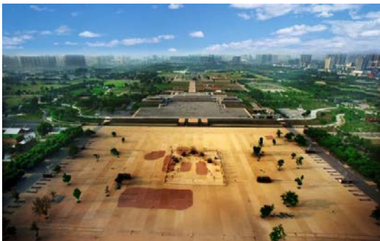
Figure 2.1: Full view of the Imperial Path and the Hanyuan Hall of the Danming Palace
