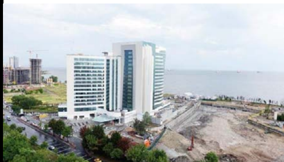
Figure 7 – Ongoing hotel construction ( http://goo.gl/ZatYtv )
