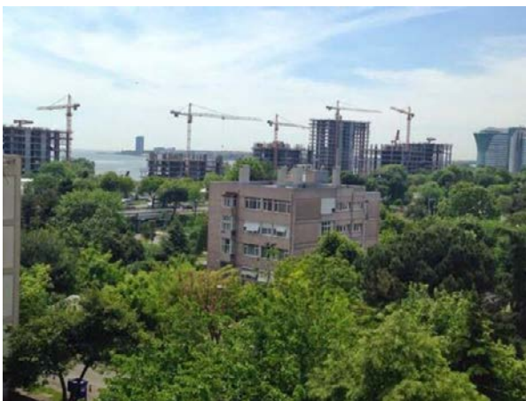
Figure 9 – Ongoing constructions in Ataköy ( http://goo.gl/YLdfLg )
