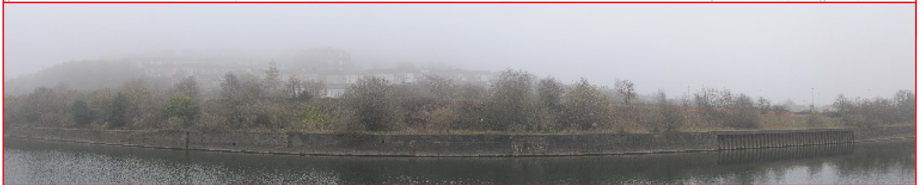
Panorama of the site (with St Thomas above in the mist) looking from the opposite bank of the River showing the mainly original river wall at which ships moored - note piled repairs to South
