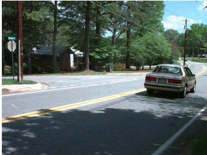
Major collector road that borders, and separates, the Tucker neighborhood from the surrounding areas.
