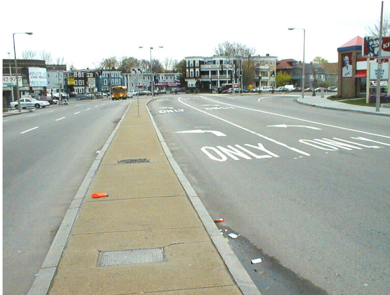
Edward Everett Square at the intersection of Columbia Road, Massachusetts Avenue, and Boston Street with its automobile oriented character: wide road pavement, loose street edge, hard-edged median, and higher-speed vehicular traffic.
