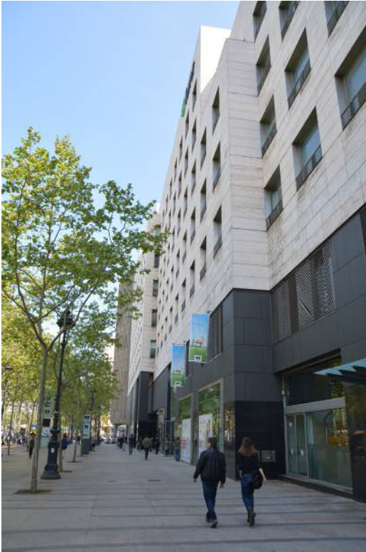
Fig. 2.2.101 View southwards towards Linkage-Entrance 1.
