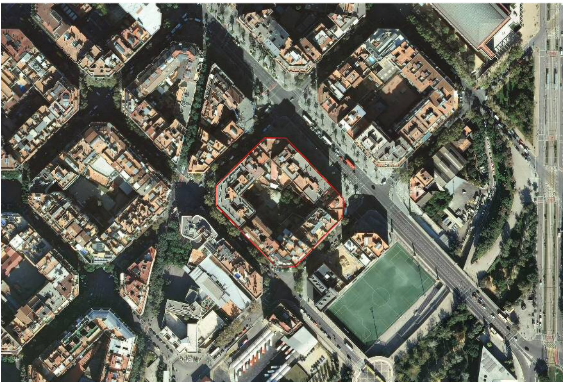
Fig. 1.2.55 Comparitive (same scale) aerial views of L'illa Diagonal (top) and Jardins de Lina Òdena (bottom).
