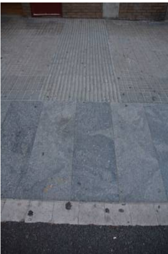
Fig. 1.2.18 Kerb allows access (from road).
