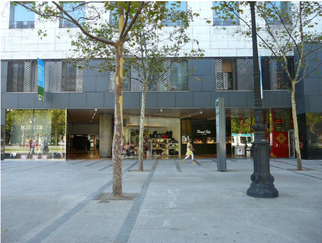
Fig. 2.2.136 View of Linkage-Entrance 3 from Avinguda Diagonal .
