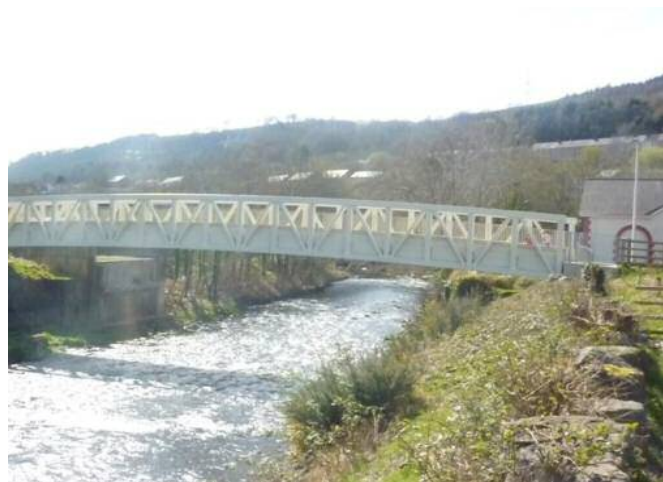
Figure 13 Bridge near Aberfan.
