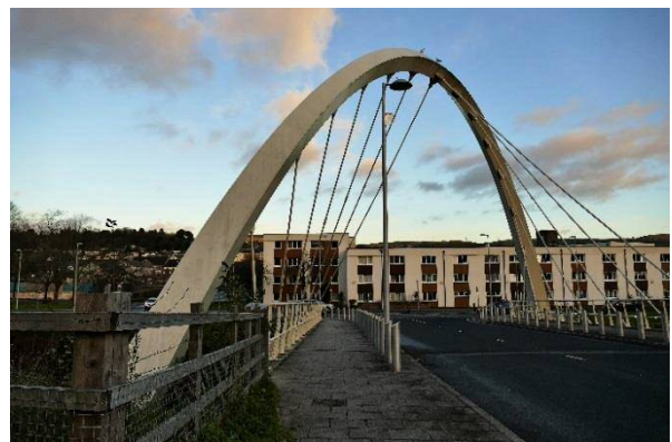
Figure 1 River Taff Bridge, Merthyr. Picture: Lesley Davies.
