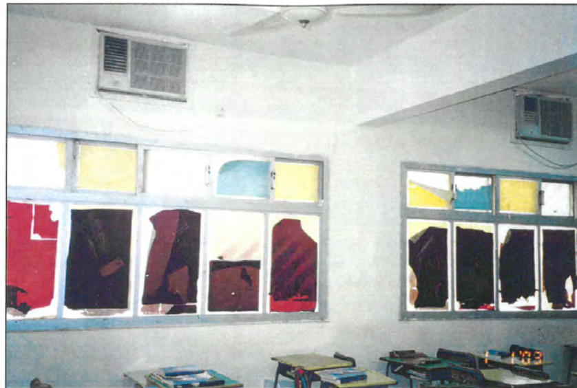
(b) Near the end of a school year, the black film is ruined because of the heat from the sun and needs to be replaced.
