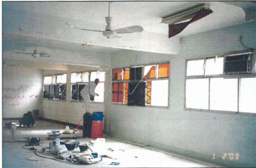
Figure 1.7: Removing the black films during annual maintenance every summer (source: Abanomi 2005).
