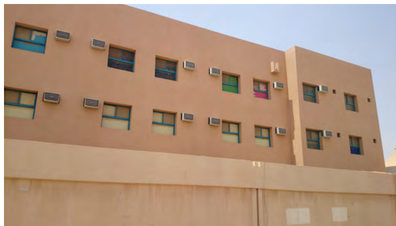
Figure 3.12: The exterior wall of school buildings showing the effect of blocking windows (taken by author 2015).
