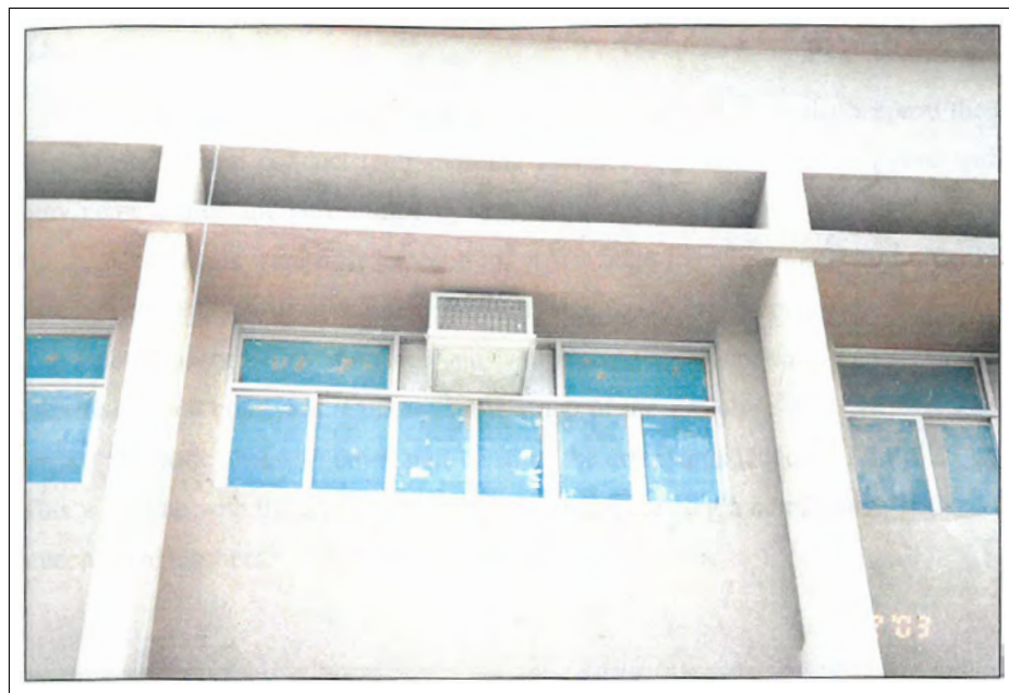
Figure 3.24: The exterior wall of schools (source: Abanomi 2005 ).
