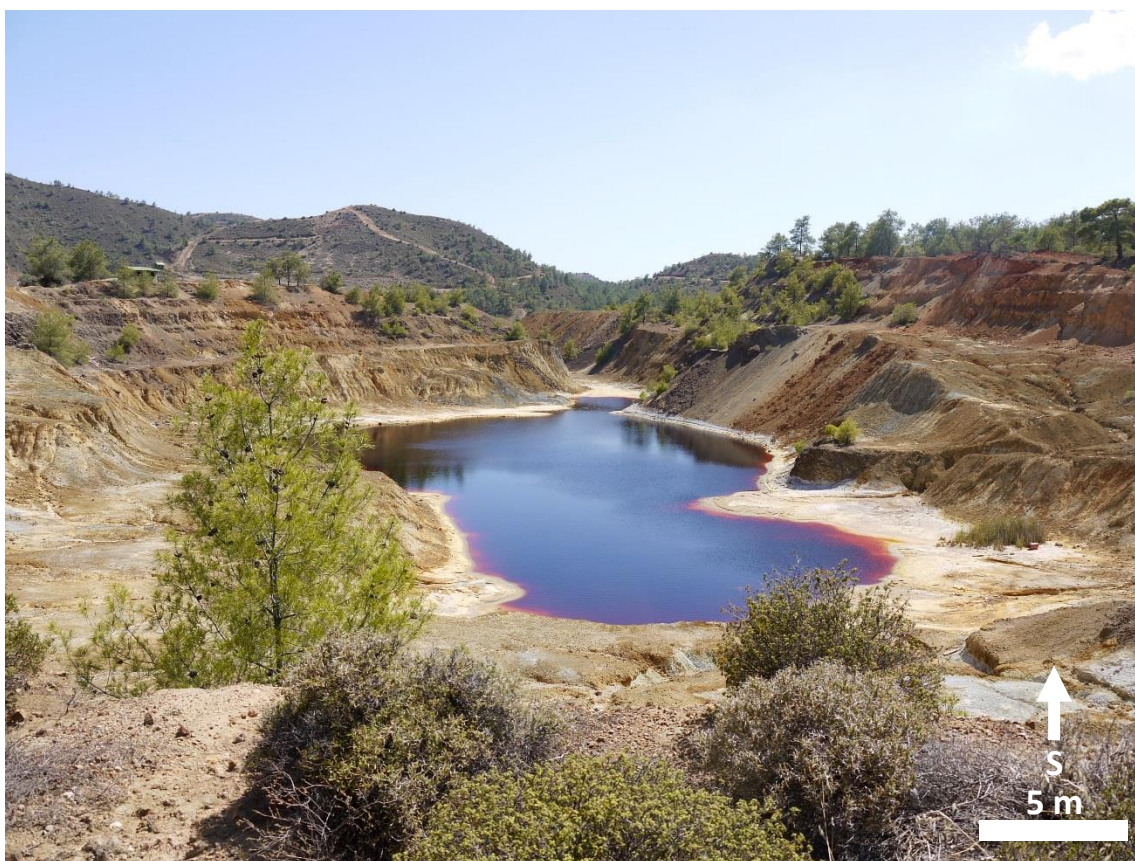
Figure A3.53: View along pit strike. Pit is 190 m long and 70 m wide at its widest point. AMD is well developed. Massive sulfide is preserved at the base of the pit.
