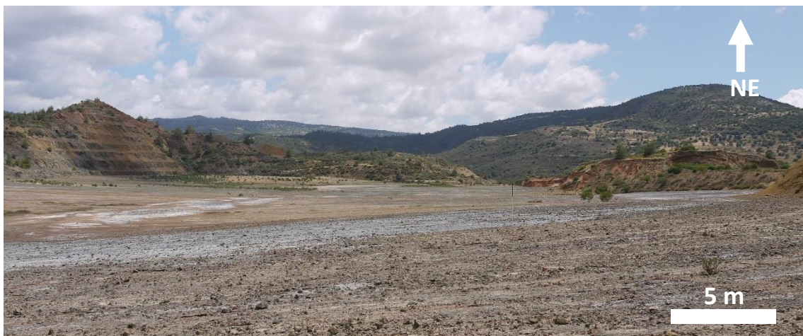
Figure A3.65: View looking E of Limni open pit. The pit has been nearly completely back filled with VMS waste. The pit is underlain by a geomembrane to stop AMD production.
