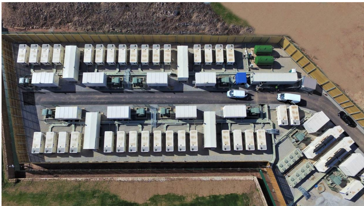
Figure 23 – An aerial shot of the 15MW lithium ion battery storage facility site in Lockleaze, North Bristol. The technology is framed as ‘zero emissions’ (FG1) by one of the founders of RADE in the focus group discussion.
