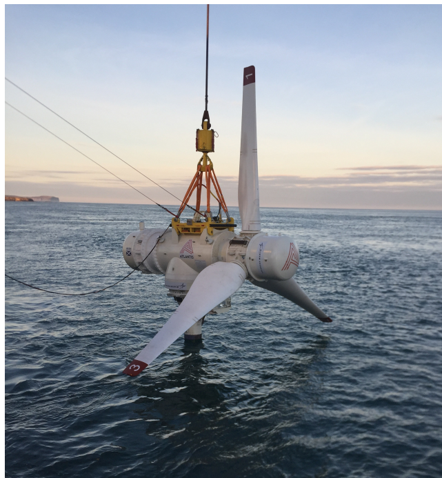
Figure 2.1: Installation of Atlantic Resources AR1500 turbine at EMEC in Orkney[23].
