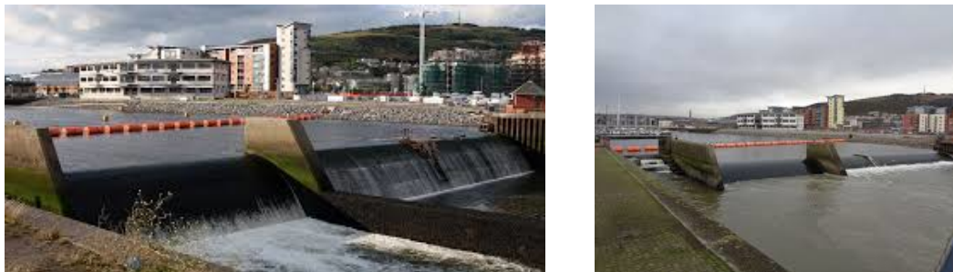
Figure 5.9: Tawe barrage and fish pass during different tidal phases
