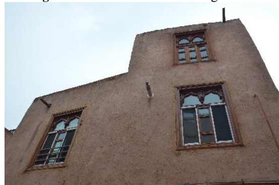
Figure 4. The thick soil wall
