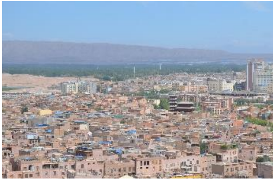
Figure 1. Low-rise and high-density buildings
