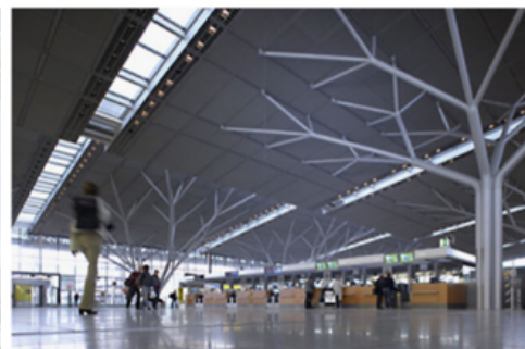
d) Structural 'trees' in Stuttgart Airport
