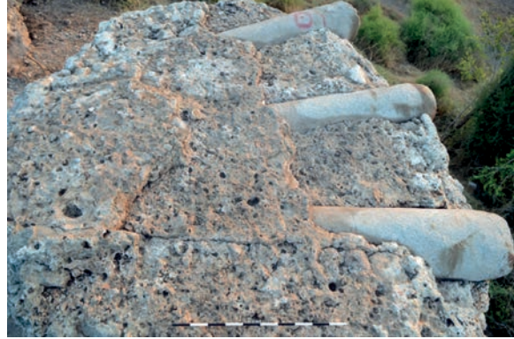
Figure 17.16. The surviving top of the Phase 3 Fatimid rounded Tower 4, showing granite through-columns (photo A14–26213)
