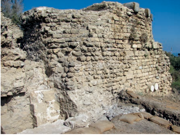
Figure 17.14. Exterior of the Phase 3 Fatimid town wall and tower (3–4) from the southeast, showing the large blocks and ghost of the Phase 7 Hellenistic Wall 44 running through it and, in the foreground, the foundation of the Phase 6 Byzantine–Fatimid wall (26, 28, 90) against which it was built; also visible are the Phase 2 (Crusader?) triangular spurs added to the Phase 3 tower (photo DP 2014)
