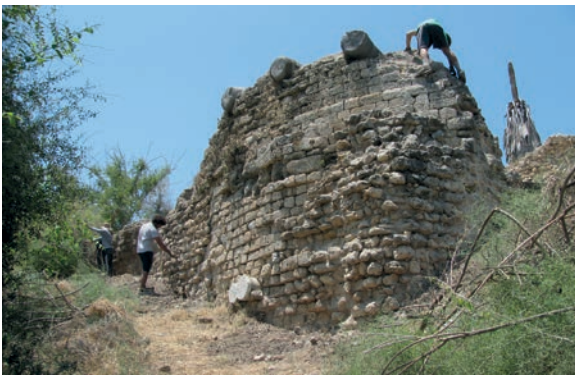
Figure 17.15. Phase 3 Fatimid rounded Tower 4 from the northeast, showing the Phase 2 triangular spurs added to square off the foundation. The original Fatimid-period ground level is indicated by the polygonal courses and plinth just above the top of the spurs (photo DP 2014)
