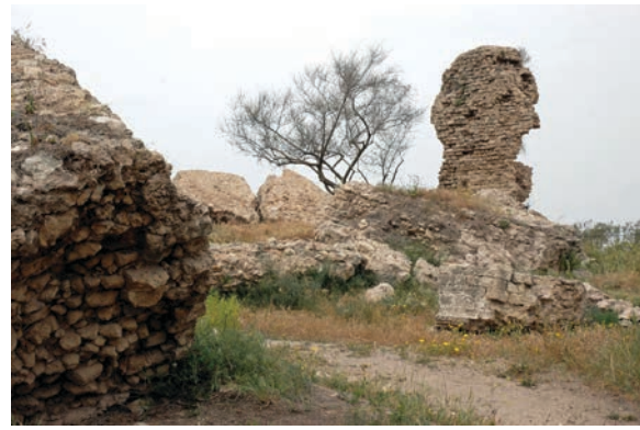
Figure 19.109. Gate tower Fragment BB2 after its collapse, with Fragments BB3 and Tower CC behind (photo Denys Pringle 2009)
