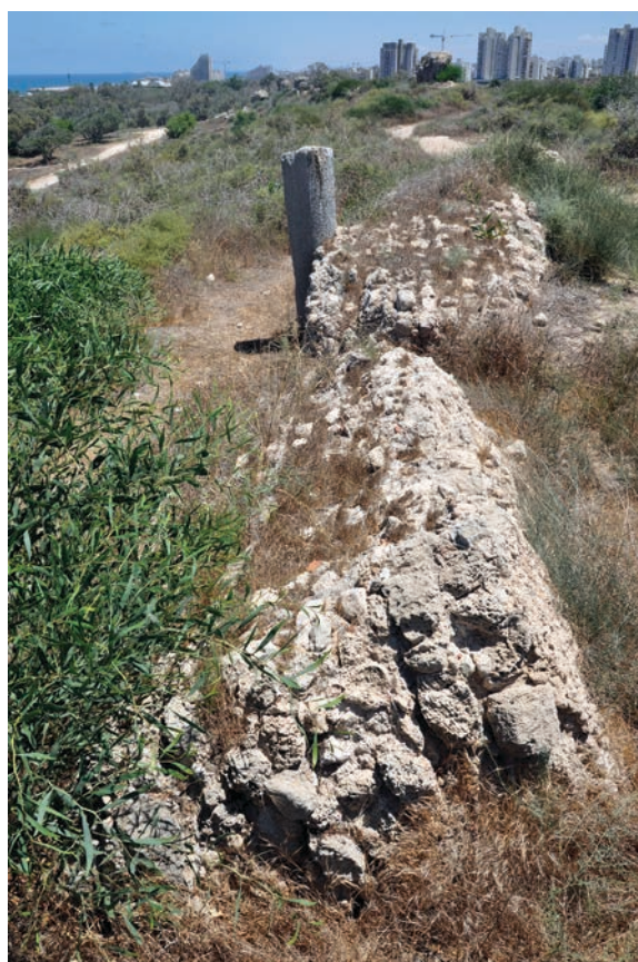
Figure 19.62. Fallen section of curtain Wall G1, from the southwest (photo Denys Pringle 2012)
