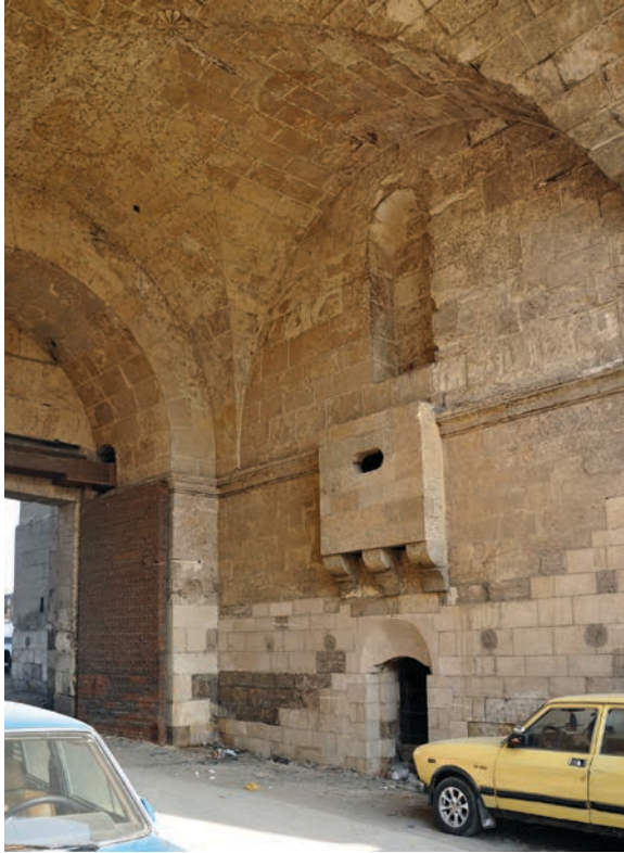
Figure 19.180. Cairo: Bab al-Futuh (1087–88), the gate passage, showing a niche above head height in the south wall (the door below it is a later insertion) (photo Denys Pringle 2011)
