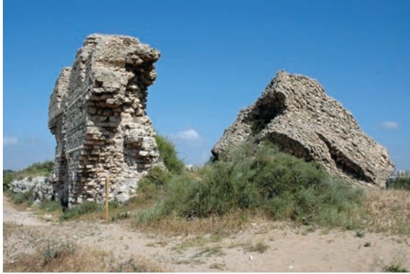
Figure 19.50. Tower E, from the west (photo Denys Pringle 2009)
