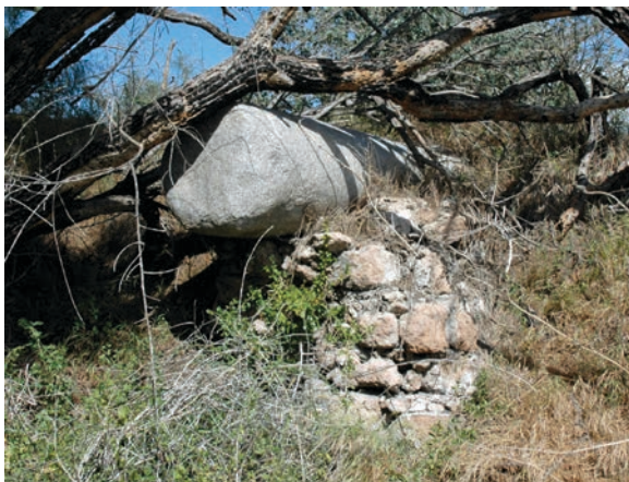
Figure 19.119. Through-column in Wall HH (photo Denys Pringle 2009)
