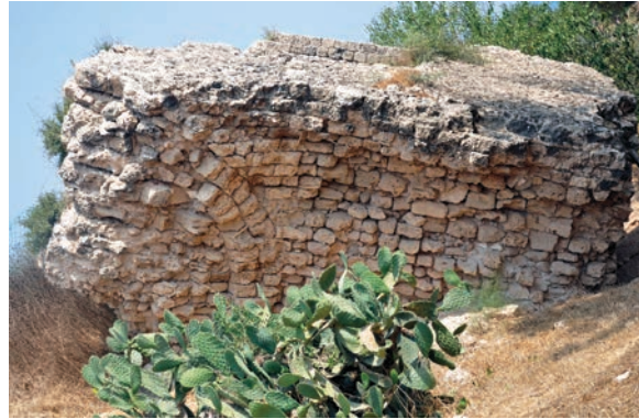
Figure 19.141. Tower R, fragment R3, east wall face showing decorative blind arch (photo Denys Pringle 2012)
