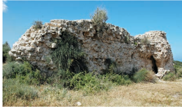
Figure 19.44. Curtain wall fragment C, from the east (photo Denys Pringle 2009)
