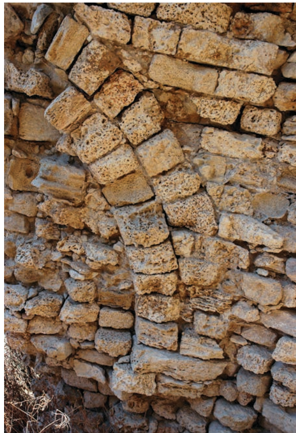
Figure 19.142. Tower R, fragment R3, detail of decorative blind arch in east wall (photo Denys Pringle 2011)
