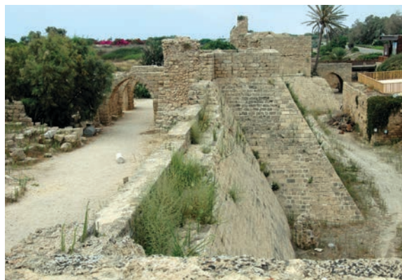
Figure 19.166. Caesarea (Qaysariyya): tower 10, incorporating an early Islamic buttress or turret, abutted by domestic buildings over the street, and enclosed by the talus and ditch of 1251–52 (photo Denys Pringle 2013)
