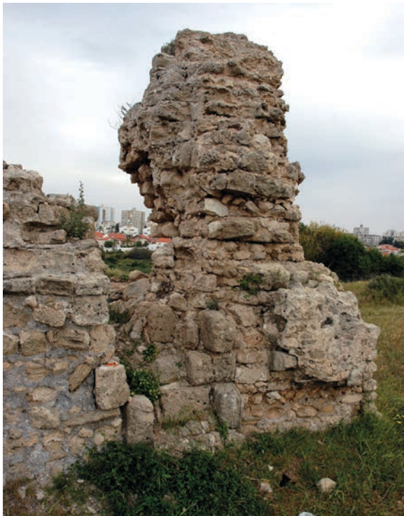
Figure 72. Fragment of Hellenistic wall incorporated into the town wall where it is abutted by Tower K (photo Denys Pringle 2009)
