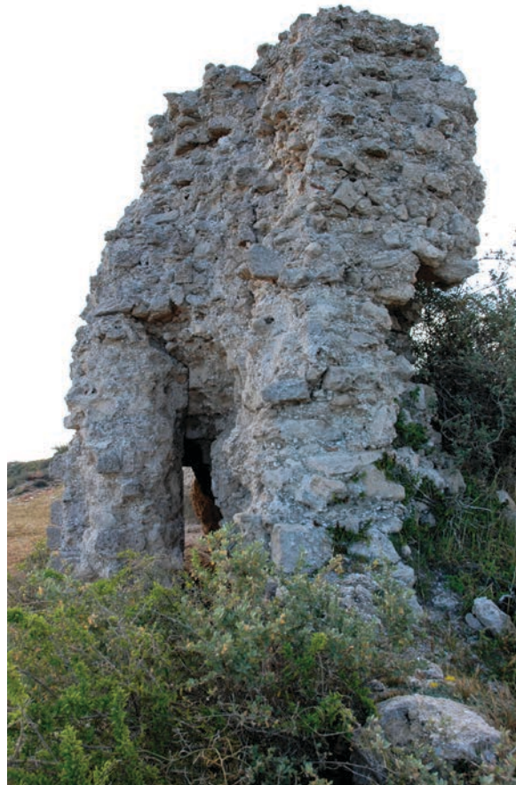
Figure 19.45. Curtain wall fragment C, from the northwest, showing Phase 1 (left) abutting and running over the top of Phase 2 (right) (photo Denys Pringle 2009)
