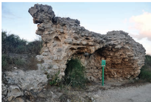
Figure 19.57. Feature F1 attached to the inside face of the town wall, viewed from the north (photo Denys Pringle 2012)
