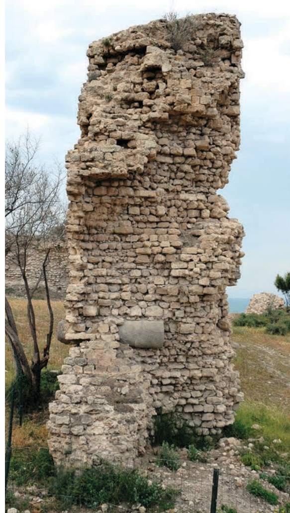
Figure 19.98. Tower CC, stump of southwest corner from east, showing basement window reveal and traces of interior wall face at first-floor level (photo Denys Pringle 2009)
