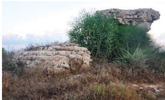
Figure 19.67. Tower or Turret H, seen from the south (photo Denys Pringle 2012)
