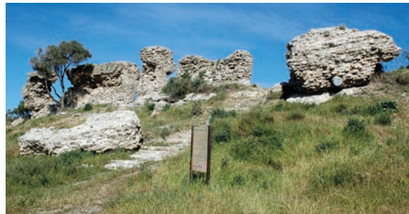
Figure 19.83. Fragments WW and VV from the west, with wall Fragment VV2 in foreground and Turret VV and Wall WW behind (photo Denys Pringle 2009)
