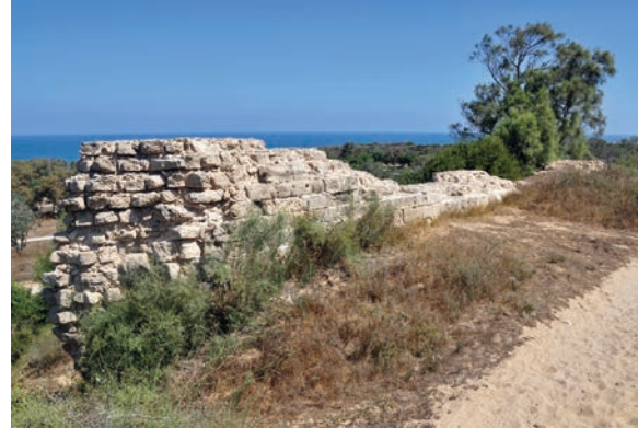
Figure 19.69. Curtain wall Fragment J, viewed from the south (photo Denys Pringle 2012)
