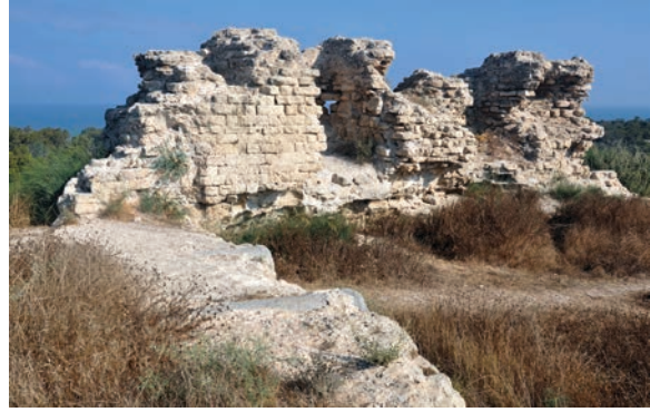
Figure 19.73. Curtain wall to the north of Tower K, east face (photo Denys Pringle 2012)
