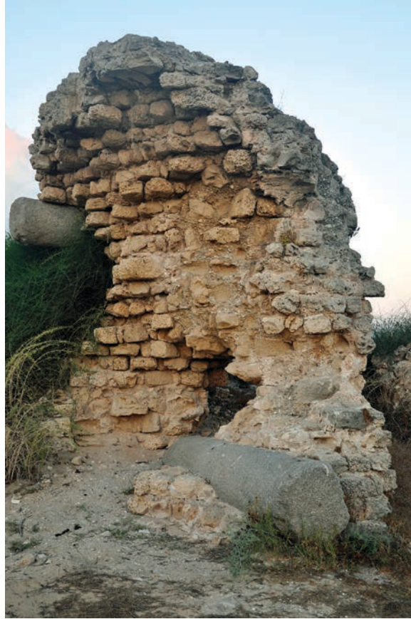
Figure 19.65. East corner of Tower or Turret H, seen from the northeast (photo Denys Pringle 2012)
