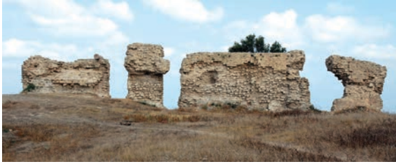
Figure 19.87. Wall WW from the east (photo Denys Pringle 2011)
