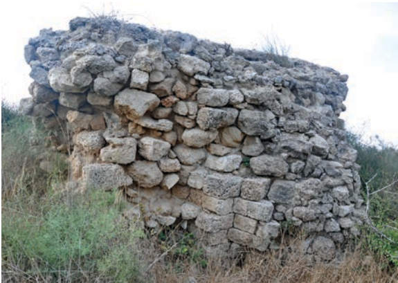
Figure 19.129. Tower Fragment AAA8 (upside down), showing internal angle (photo Denys Pringle 2012)
