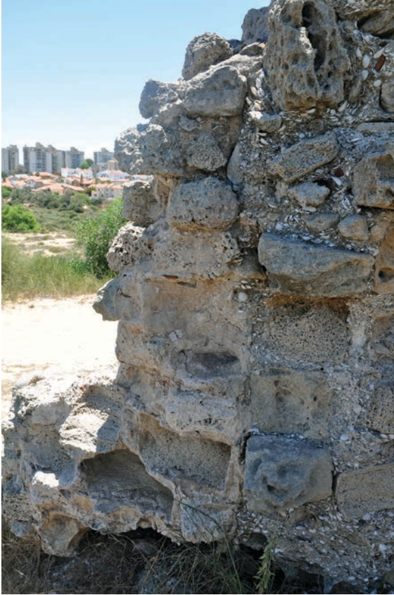
Figure 19.64. Detail of the west side of H, showing the Phase 2 shelly-mortared masonry (right) intersected by the Phase 1 addition (left) (photo Denys Pringle 2012)
