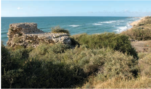
Figure 19.41. Fragment of curtain Wall JJ3, with view along shore to the north (photo Denys Pringle 2009)
