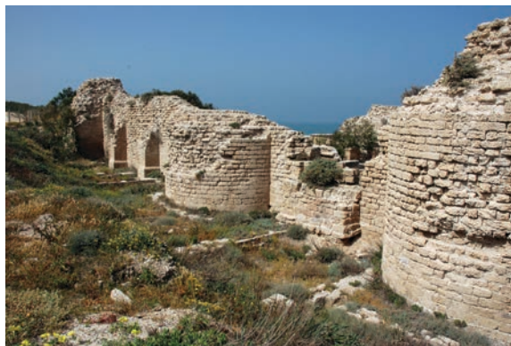
Figure 19.163. Mahuz Azdud (Minat al-Qal'a, Ashdod Yam): Umayyad fort, east wall and blocked gate (photo Denys Pringle 2009)
