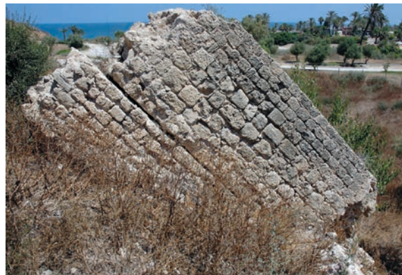
Figure 19.138. Tower R, fragment R2, interior wall face (photo Denys Pringle 2011)
