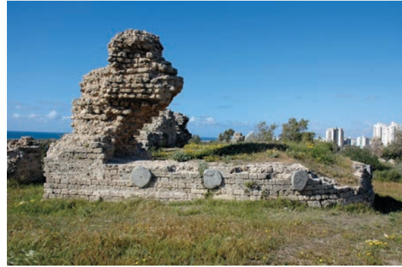
Figure 19.78. Tower K, from the south (photo Denys Pringle 2009)
