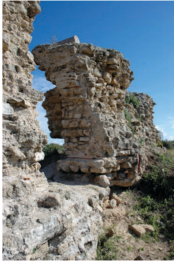
Figure 19.92. The north end of the southern block of wall WW from the north, showing the exposed filled-in cistern WW2 and overflow pipe (photo Denys Pringle 2012)
