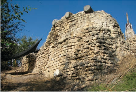
Figure 19.124. Tower FF from the northeast (photo Denys Pringle 2014)
