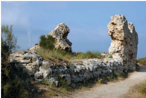
Figure 19.51. Tower E, from the northeast (photo Denys Pringle 2011)
