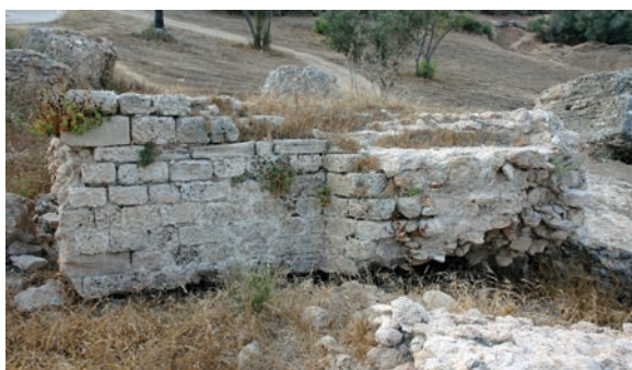
Figure 19.111. Gate tower Fragment BB2 (upside down), showing the outer gate passage and remains of the door jamb and portcullis slot (photo Denys Pringle 2011)
