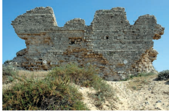
Figure 19.52. Tower E, rear wall overlying the earlier curtain wall, seen from the northwest (photo Denys Pringle 2009)
