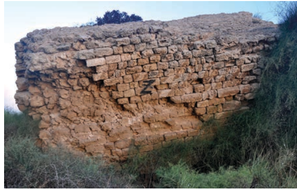
Figure 19.54. Tower E, detached fragment, east face (photo Denys Pringle 2012)
