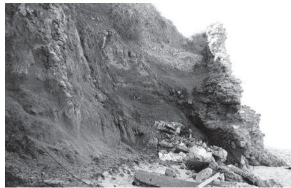
Figure 19.31. Sea wall A and cliff section behind it (photo Denys Pringle 1983)
