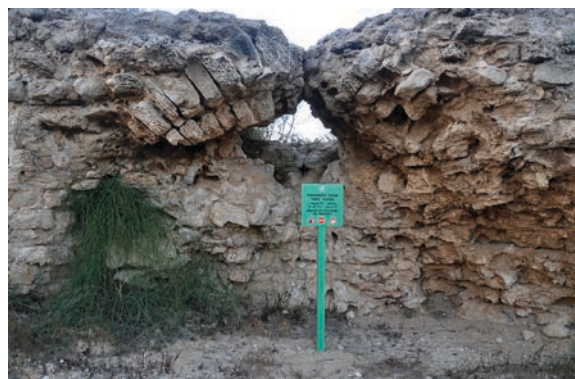
Figure 19.58. The arched recess in Feature F1, attached to the inside face of the town wall (photo Denys Pringle 2012)
