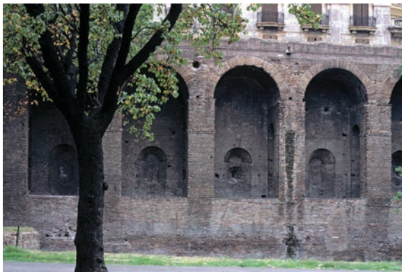
Figure 19.154. Rome: arcaded addition made by Maxentius (306–12) to the city wall near Porta San Giovanni (photo Denys Pringle 1982)
