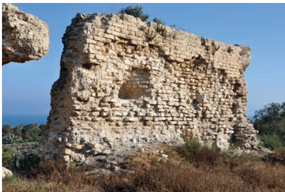
Figure 19.93. The east face of block WW6, representing mainly Phase 1 (Umayyad/Abbasid) work built off the Phase 2 (Byzantine) foundation (photo Denys Pringle 2009)
