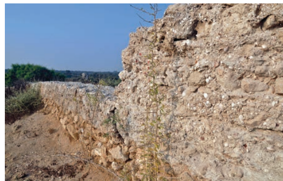
Figure 19.147. Medieval town wall (S) overlying wall of the Hellenistic period (photo Denys Pringle 2012)
