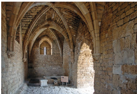
Figure 19.165. Caesarea (Qaysariyya): the east gate (1251–52), incorporating the two towers of the early Islamic gate, whose faces are represented by the areas of larger ashlar masonry on the right-hand side of the gate passage (photo Denys Pringle 2013)
