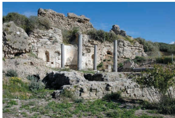
Figure 19.76. Byzantine and later chapel whose chevet forms part of a retaining wall supporting the rampart behind the town wall (photo Denys Pringle 2009)
