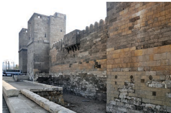
Figure 19.178. Cairo: the north wall of Badr al-Jamali (1087–92), looking east toward Bab al-Nasir. Note the through-columns near the base of the walls and towers (photo Denys Pringle 2011)
