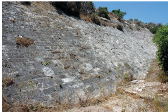
Figure 19.144. The base of the masonry Talus (RR), showing the change from granite to marble through-columns (photo Denys Pringle 2008)
