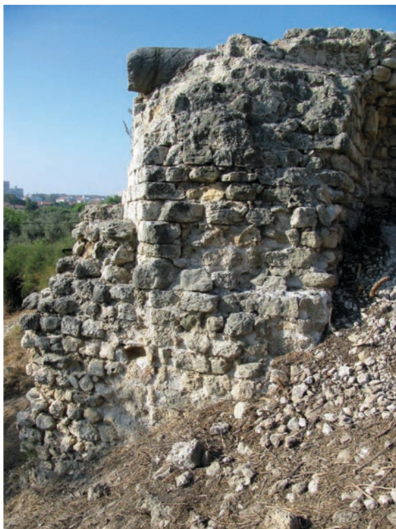
Figure 19.126. Tower FF, from the north, showing the Phase 2 spur running against the curving Phase 3 ashlar face and the squaring off of the north side of the tower (photo Denys Pringle 2014)
