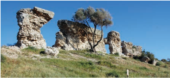
Figure 19.88. Wall WW from the northwest (photo Denys Pringle 2009)
