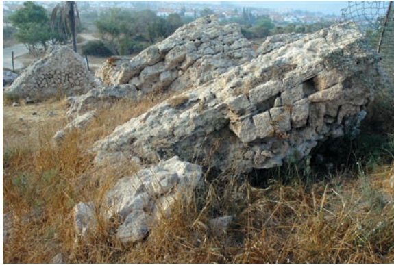
Figure 19.117. Gate tower Fragment BB4, segmental arch over the inner end of the gate passage, with Fragments BB3 and BB2 (stump) behind (photo Denys Pringle 2011)
