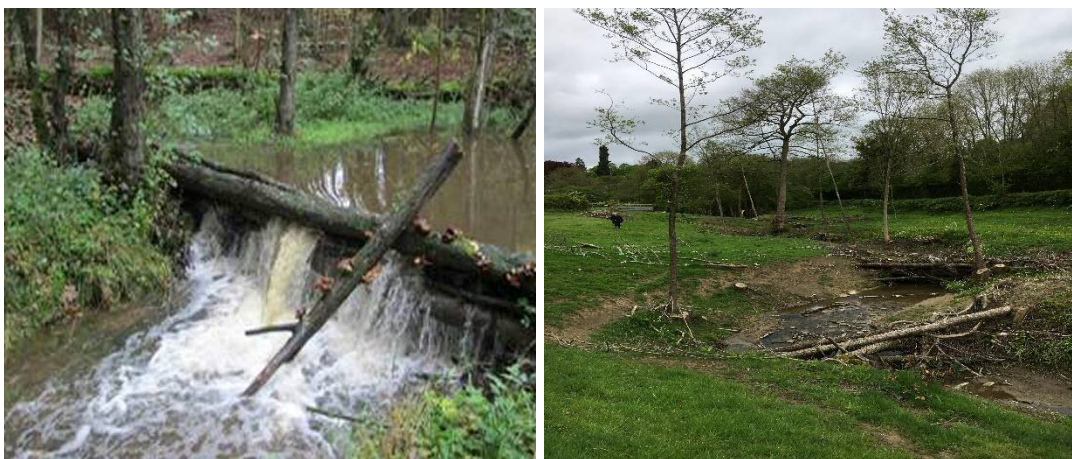
Figure 1.2. Field photographs of WDD (left) depicting backwater rise upstream of the dam (Source: Slow The Flow Calderdale, 2019) and (right) a series of WDD on Wilde Brook, part of ‘Shropshire Slow the Flow’.
