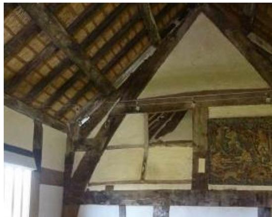
Figure 2. Internally exposed frame.
