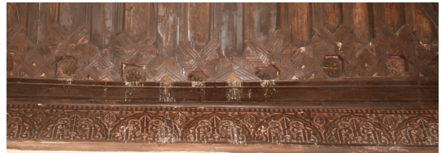
Fig. 18 North-east slope of the inner timber frame that covers the mosque's praying space. The eight-point stars at the lower end of the central rafters evidence a profound deformation due to their support's failure at the level of the wall plate. (Wulff 2012)
