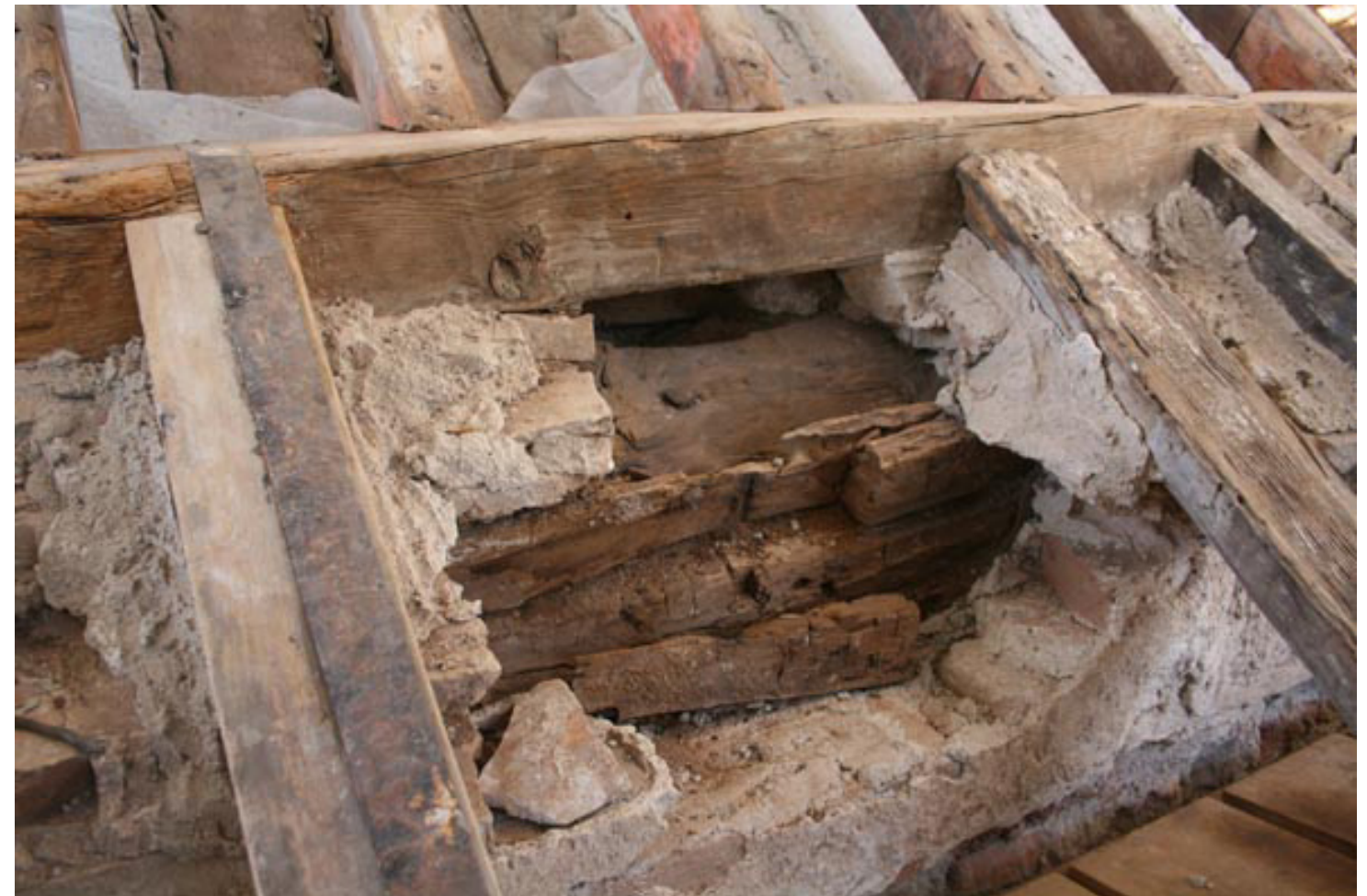
Fig. 49 Remains of the original Nasrid timber wall plate, with an unusual shape compared to its mudéjar equivalents (Artyco 2015)
