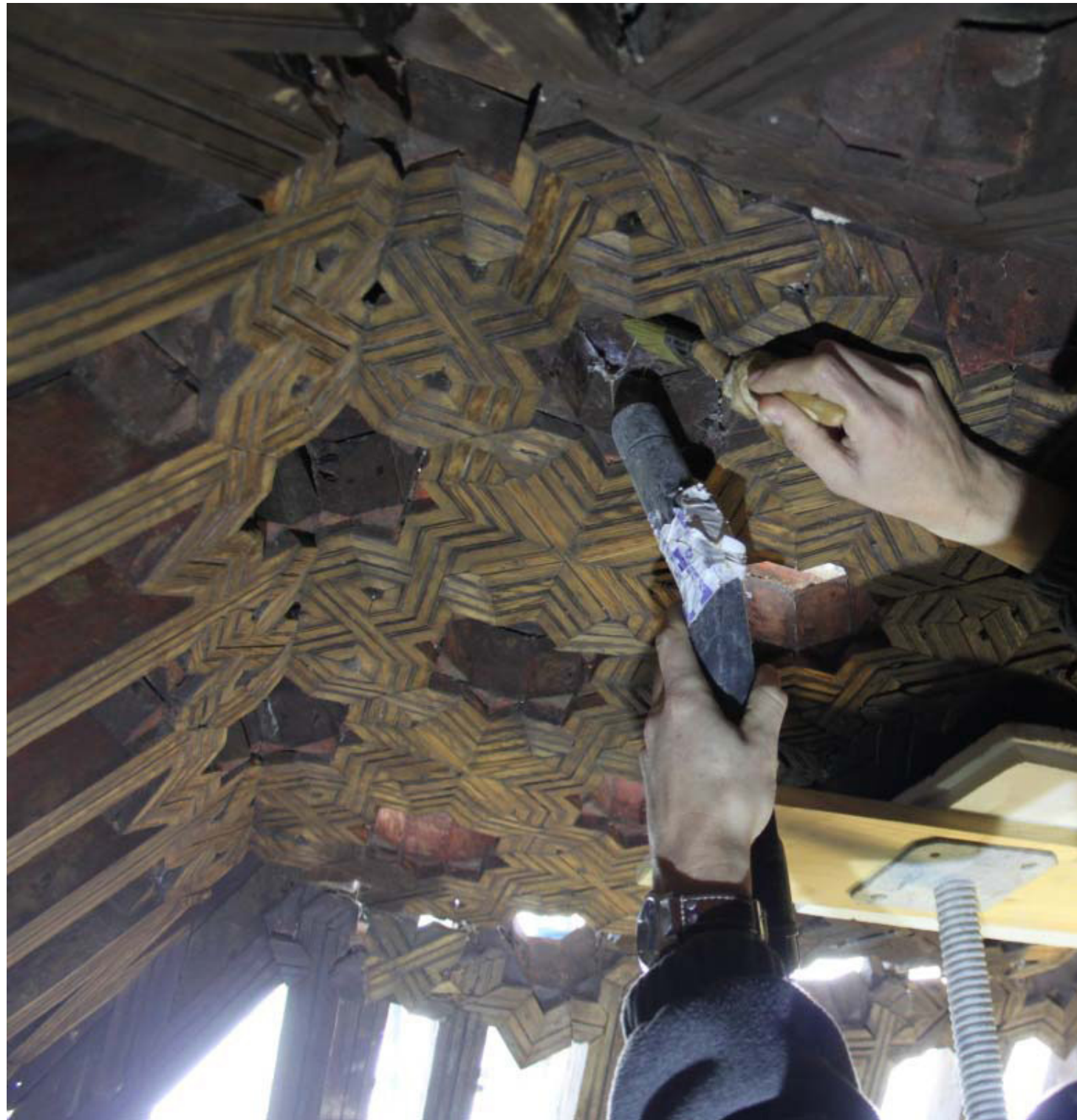
Fig.28 Preliminary superficial cleaning of dust and organic remains with vacuum and brush.
