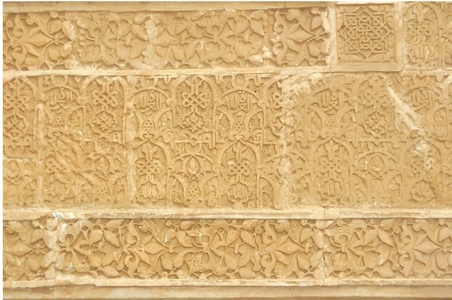
Fig. 15 Restored plaster panels from the 1846 intervention, including epigraphs and vegetal decorations that frame the windows of the south-west elevation, kept by Torres Balbás in his 1930 intervention (Wulff 2012)
