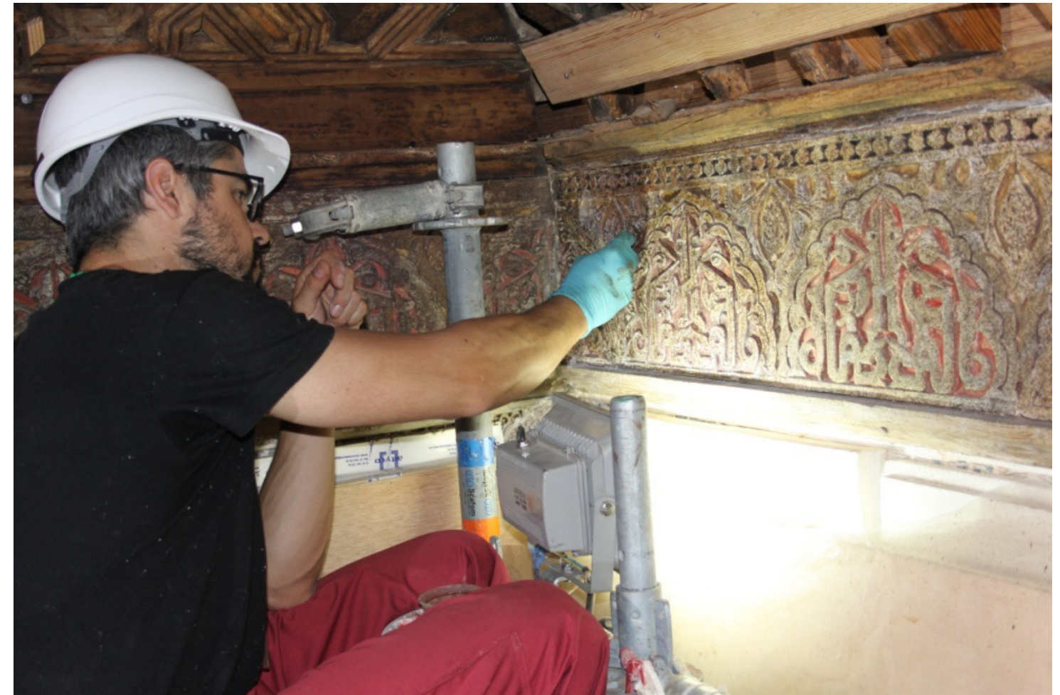
Fig.33 1846 restored plaster frieze chromatic reintegration with the other three Nasrid wooden friezes
