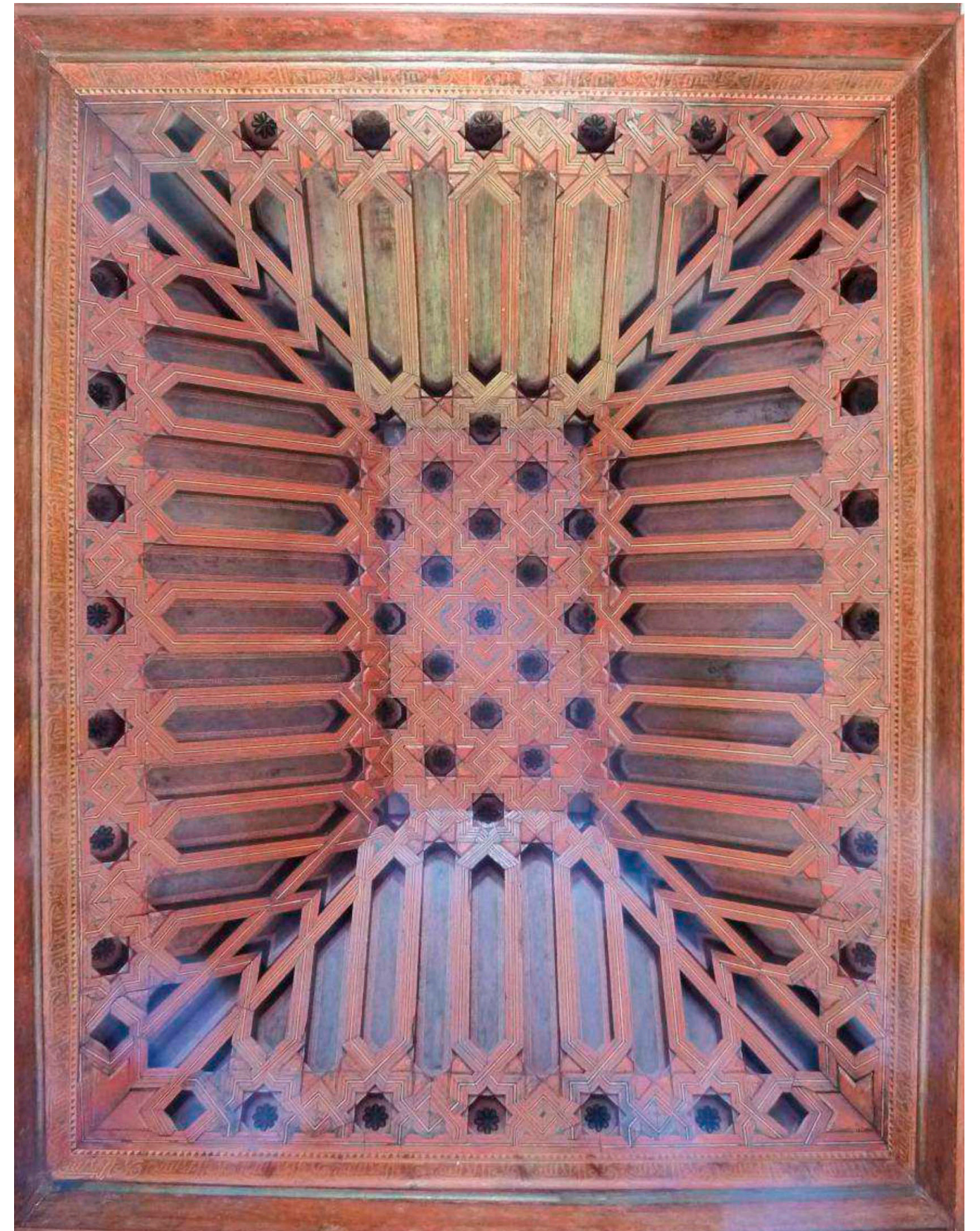
Fig. 56 The Paintings' House timber framework, also in the Partal Palace, attributed to Yusuf I (1333-1354). The regular eight-point star decorative pattern of its upper horizontal plane ( almizate ) is almost identical to the first version of the Oratory's timber framework, as shown in Fig. 55 (Wulff 2012).
