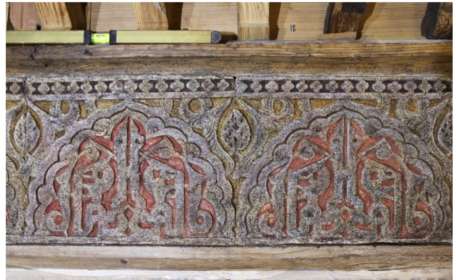
Fig.34 Cleaning of the last coating on the wooden frieze applied by the 1930 intervention with a laser of 1064 nm wavelength
