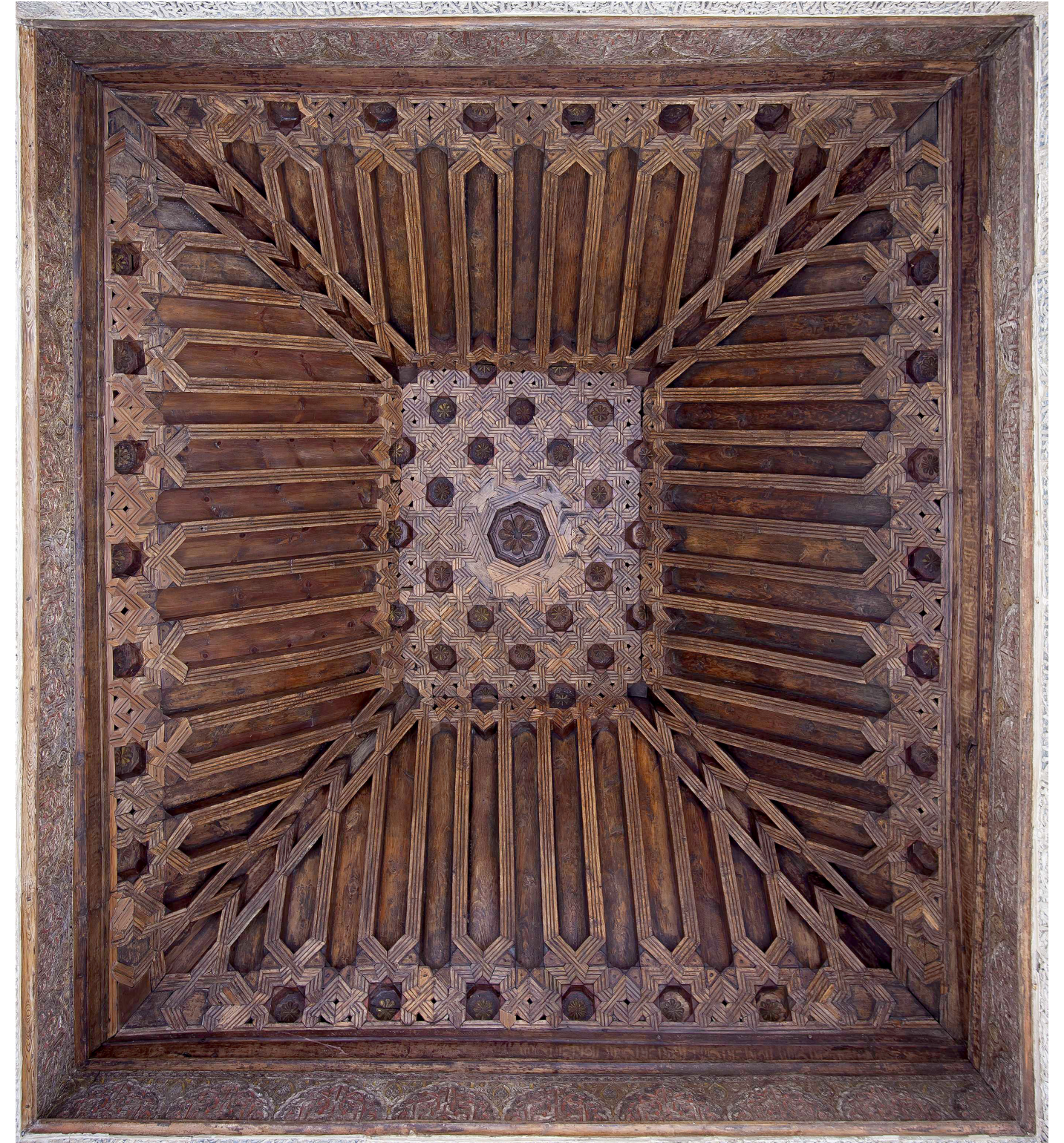
Fig. 47 The Oratory's timber framework after the 2013-2015 restoration. (Alhambra Council 2015)
