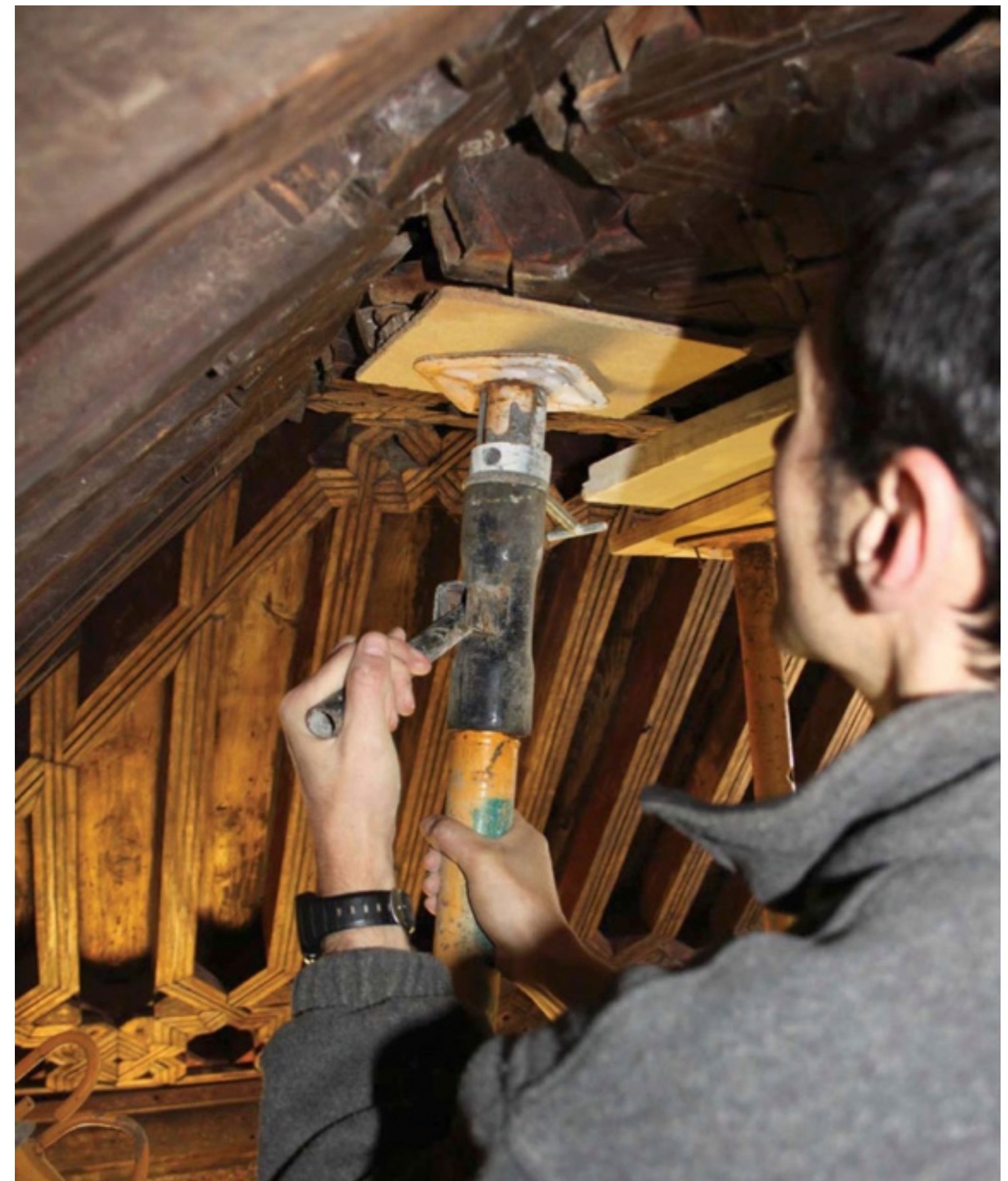
Fig.27 ( left ) Replacement of a section of the original Nasrid timber wall plate
