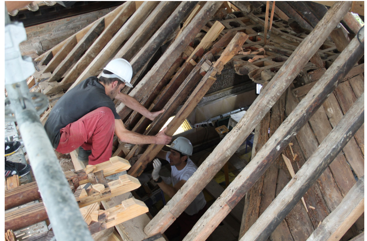
Fig.30 Assembling of the rafters of the inner timber framework to the collar ties and the wall plate. Their new added prostheses are apparent on their upper end.
