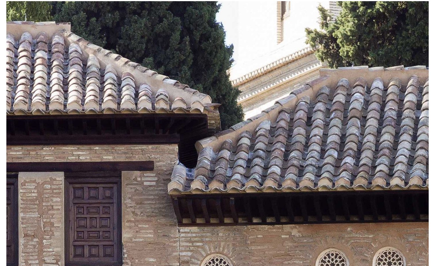
Fig. 17 The Oratory and the House of Astasio's hipped roofs encounter, pouring the rainwater off the north-west wall of the House of Astasio. (Alhambra Council 2015)
