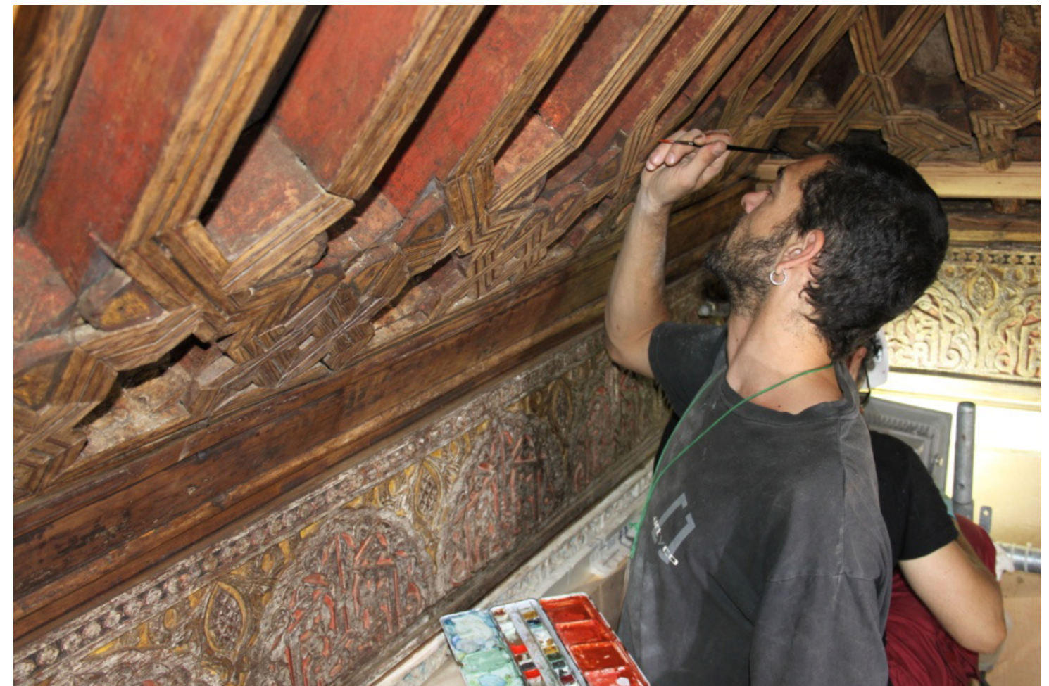
Fig.30 Assembling of the rafters of the inner timber framework to the collar ties and the wall plate. Their new added prostheses are apparent on their upper end.
