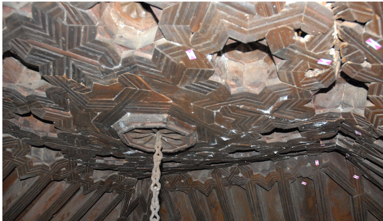
Fig. 16 Profound warping on the horizontal plane on the decorated timber frame ( almizate ), due to the inadequate overload of the roof (Wulff 2012)
