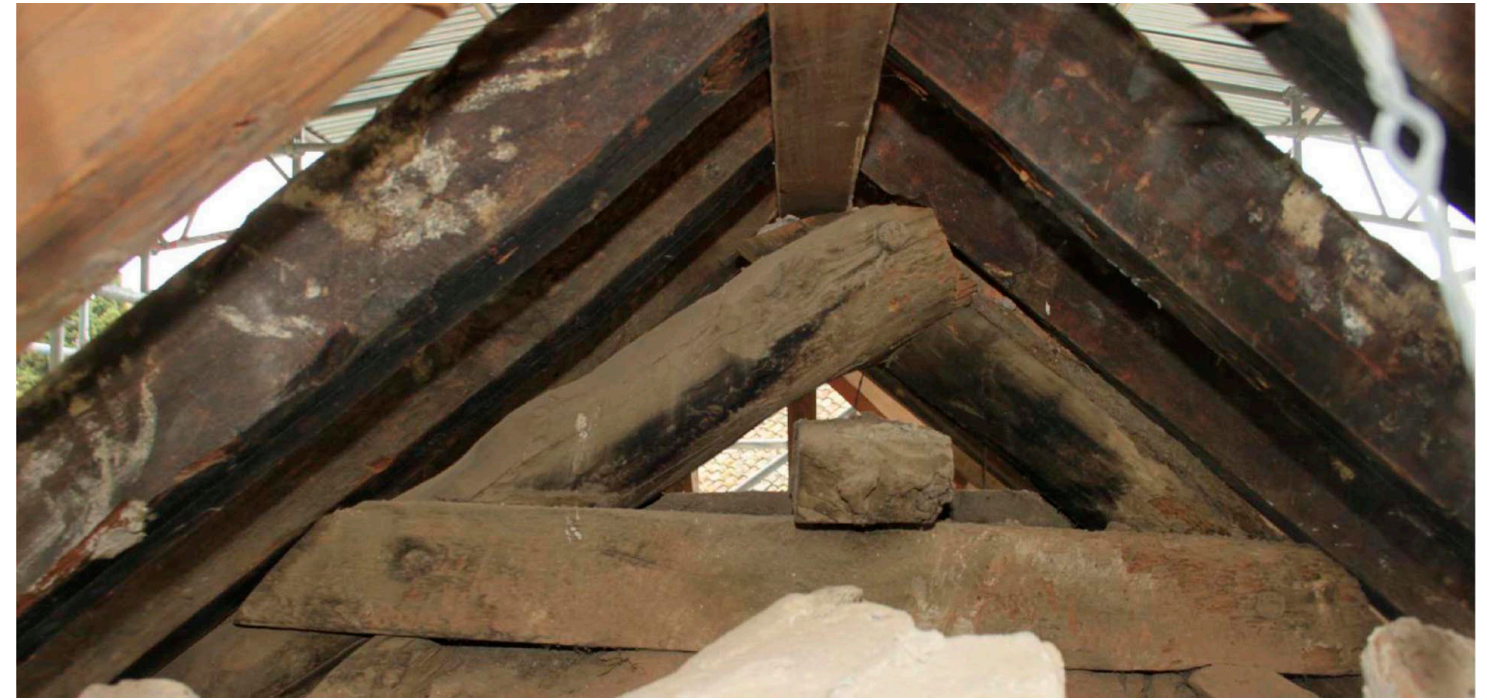
Fig. 48 Remains of the original Nasrid upper roof's structure: two rafters and a false double collar tie (Artyco 2015). These have been dated by a Carbon-14 test between 1290 and 1400 with a 95.4% probability (Uppsala Universitet 2014)
