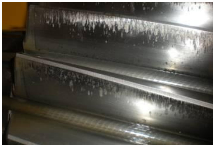
Figure 1.7 Scuffing failure in helical gear teeth at their tips. Source: Courtesy of Design Unit, Newcastle University.
