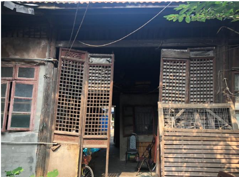
Figure 1.1 A historic house lack of maintenance
