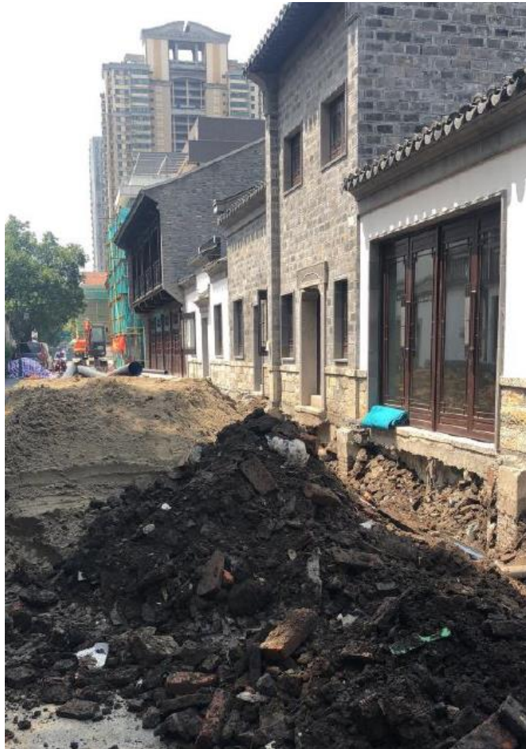
Figure 7.3 Buildings under reconstruction in Pingshijie neighbourhood
