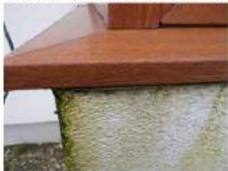
Porch - Taken Dec. 2018 EWI identifying the dry bond allowing water ingress and a large growth
