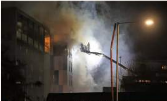
Images from after the fire show that much of the cladding on the top two floors has been burned away or has fallen off. Firefighters tackle Friday's blaze at The Cube in Bolton. Photograph: Peter Byrne/PA
