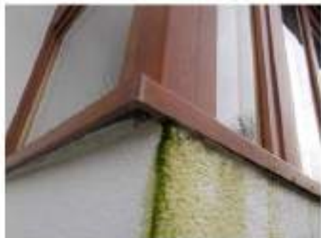
Porch - Taken Dec. 2018 EWI identifying the dry bond allowing water ingress and a large growth
