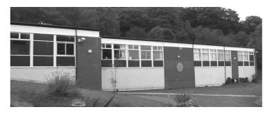
Figure 4: Edwardsville Primary School, built in the early 1970's. Example of single storey, poorly insulated school building common to communities across Britain.
