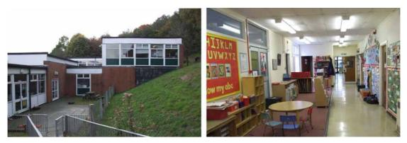
**Figure 52**: North façade of the school – external space is a 'frost pocket' to classrooms trapping cool air that sinks down the hillside
