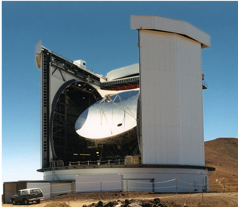
Figure 1.10. The James Clark Maxwell telescope with the dome open, showing the 15m dish. Image credit: East Asian Observatory
