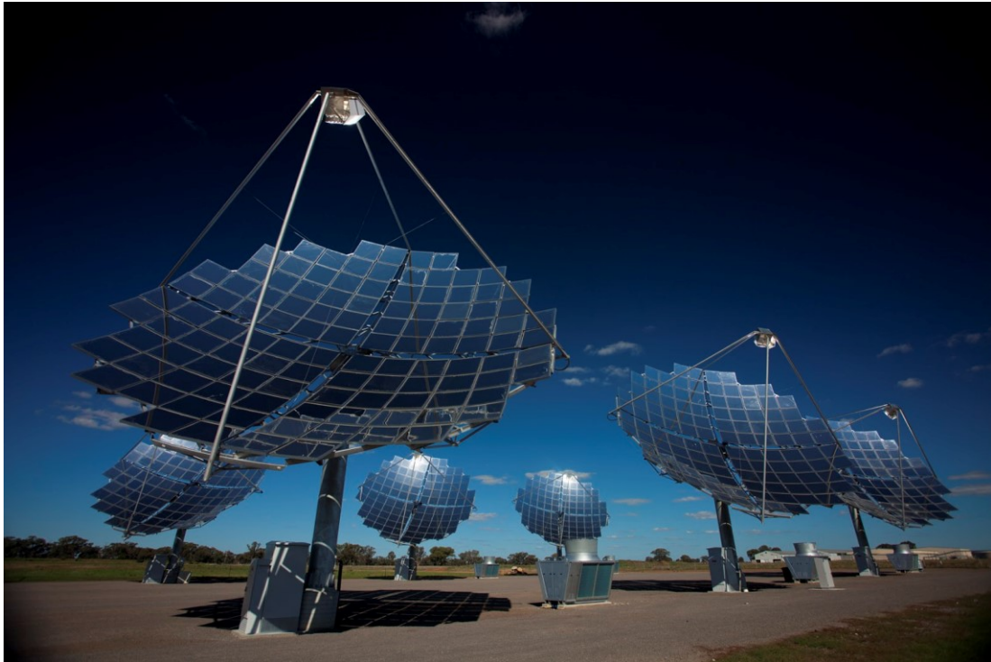
Figure 2.15: 1.5 MW concentrated PV solar dish concentrator in Mildura, Australia [81].
