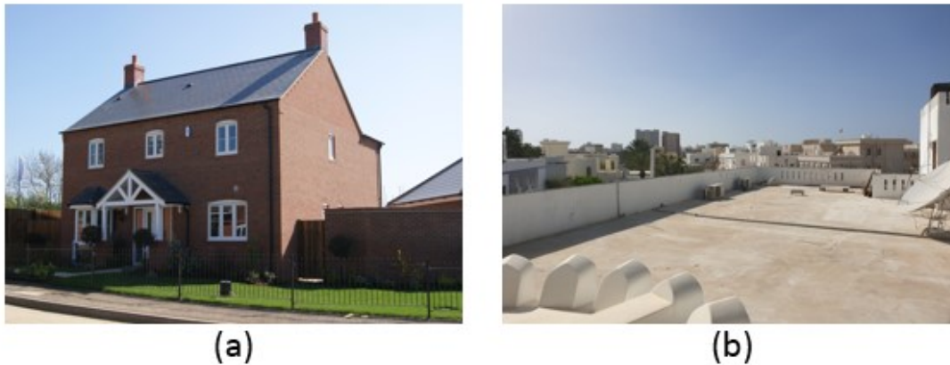
Figure 2.38: Rooftop architecture for: (a) the UK, and (b) Oman.
