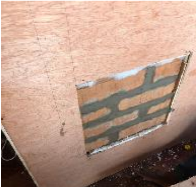
Figure 3.17: External view of the in-situ thermal test
