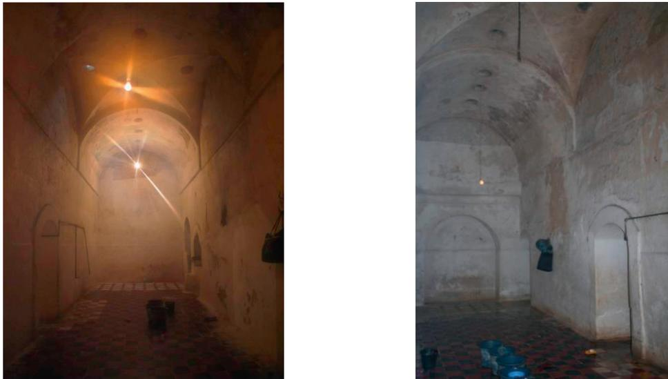
Figure 3: The hot room of hammām Seffarine in Fez in 2006 when the roof openings were blocked (photo by Dr Magda Sibley)
