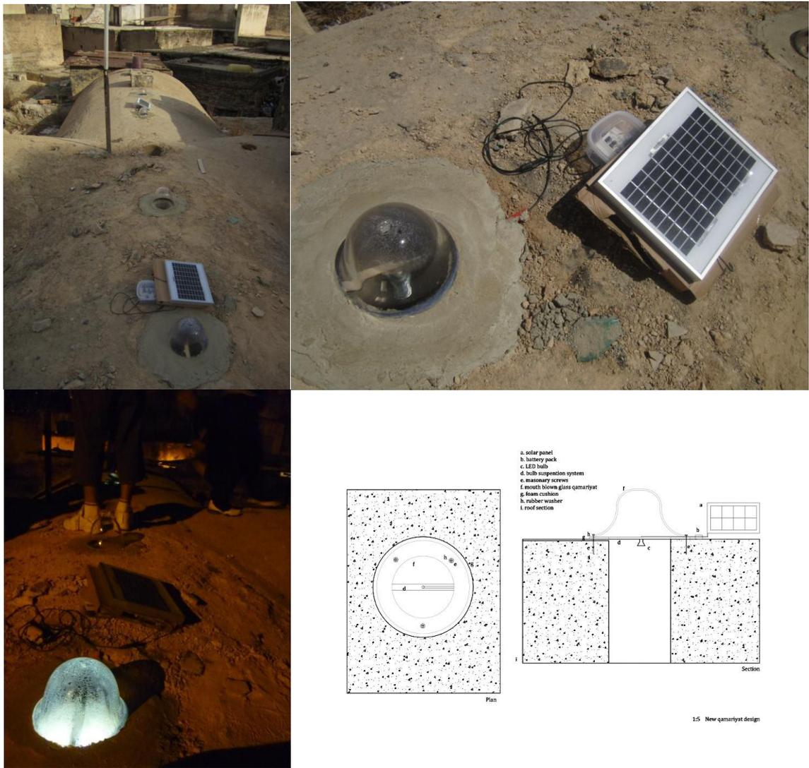
Figure 5: Day and night view of the glass bulbs installed on the roof on the hot room of hammām Seffarine in September 2012(top and bottom left) and plan and section of the glass bulb installation (bottom right)
