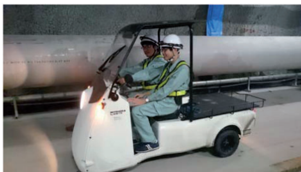
Fig. 10. Each worker is equipped with a helmet, work clothes, reflective vest, and headlight for work inside the tunnel. Small electric carts are used for the 3 km transport from the central area to the end station.
