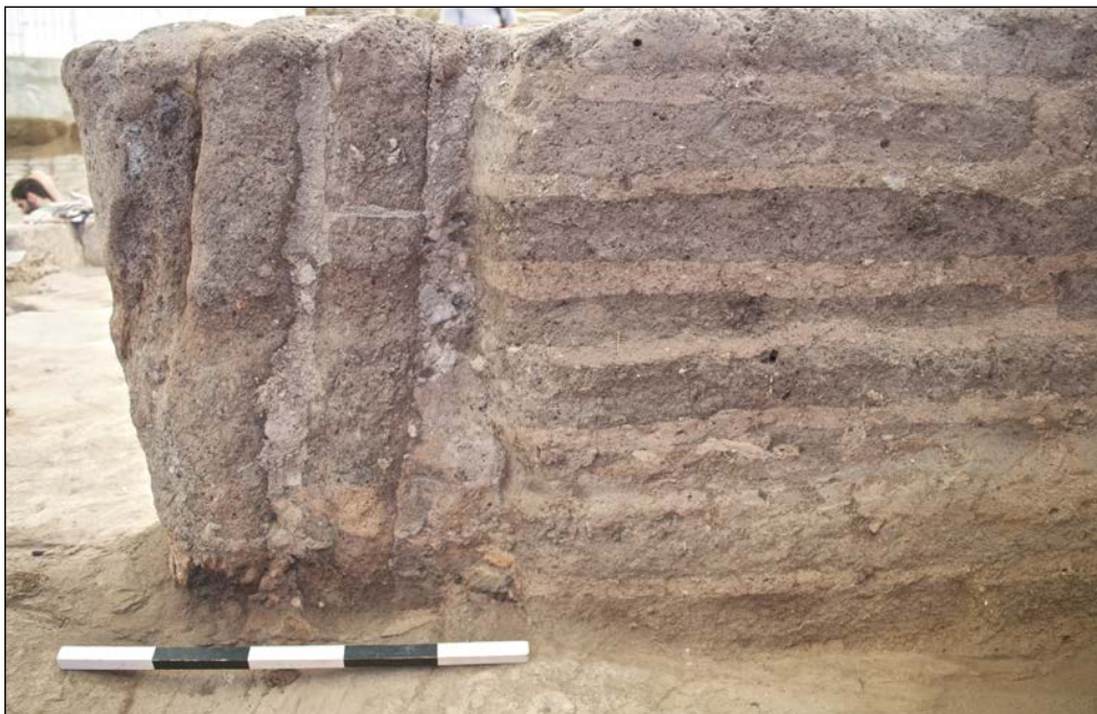
Figure 3.22. South-facing side of partition wall extension F.7403 with vertical bricks (north facing, Photo: Justine Issavi).
