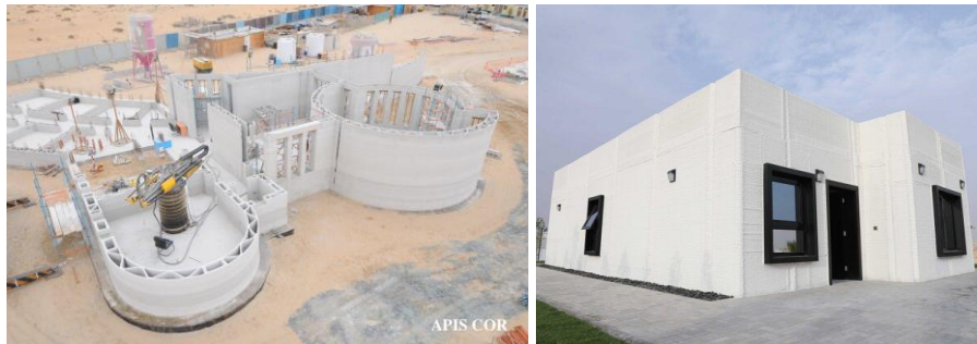
Figure 1: Notable examples of 3DP concrete buildings: (a) Two-storey office building in Dubai constructed by Apis Cor (image credit: Apis Cor), and (b) House in Saudi Arabia constructed by CyBe (image credit: CyBe).
