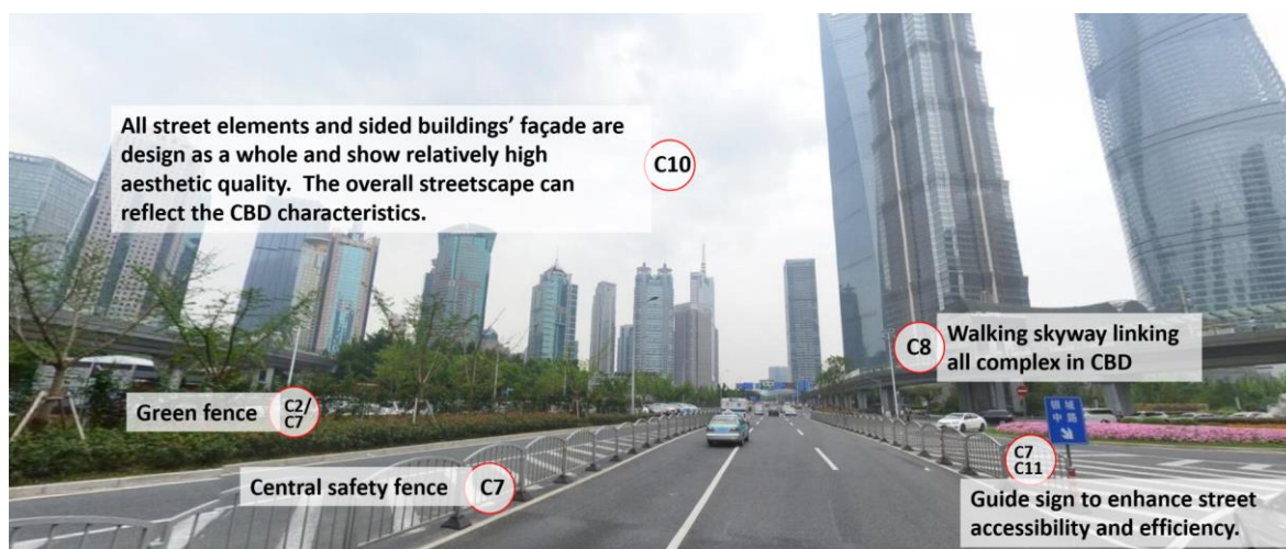
Figure II. 1: Evaluation Illustration on On-Site Photo of C2-6 (Century Avenue)
