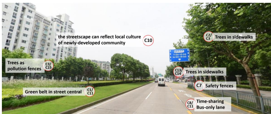
Figure Y. 1: Evaluation Illustration on On-Site Photo of M9-1 (Zhangyang Rd)
