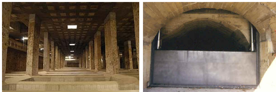
Figure 2.9 Elements of the sewer system (tanks and sluices) (CLABSA 2010).
