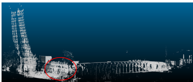
Figure 1. Pointcloud of the Minakshi Sundareshvara Temple, Madurai showing the Pudhu Mandapam from TLS (3 scans) made in 2018 looking East (West front indicated by the circle)
