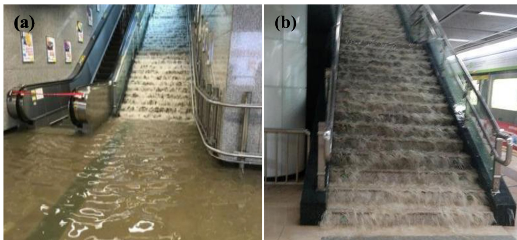
43 44 Figure 1: Metro station inundated during urban flooding. (a) Changpan station flooded on 10th May, 2016 in Guangzhou (Lyu et al. 2016); (b) 45 Zhongnan station flooded on 6th July, 2016 in Wuhan. 46 47
