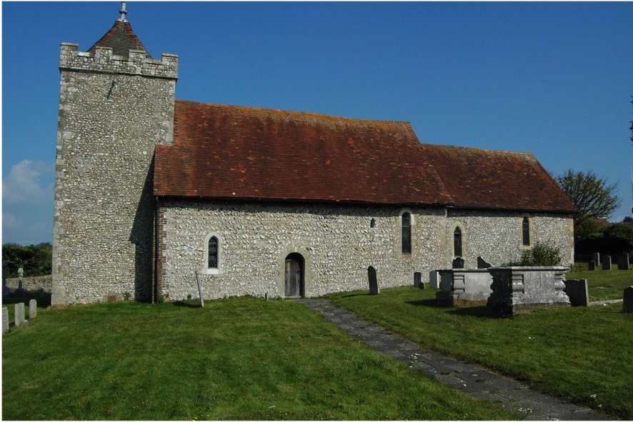
Fig. 7 The church of St Helen, Hangleton, viewed from the south. The tower was added in the early thirteenth century and the chancel (to the right) was re-built around 1300 (photograph: Ben Jervis)
