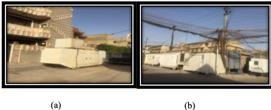
**Figure 1-10 Private diesel generators connected (a) to a single house (b) to the community with private wires**
