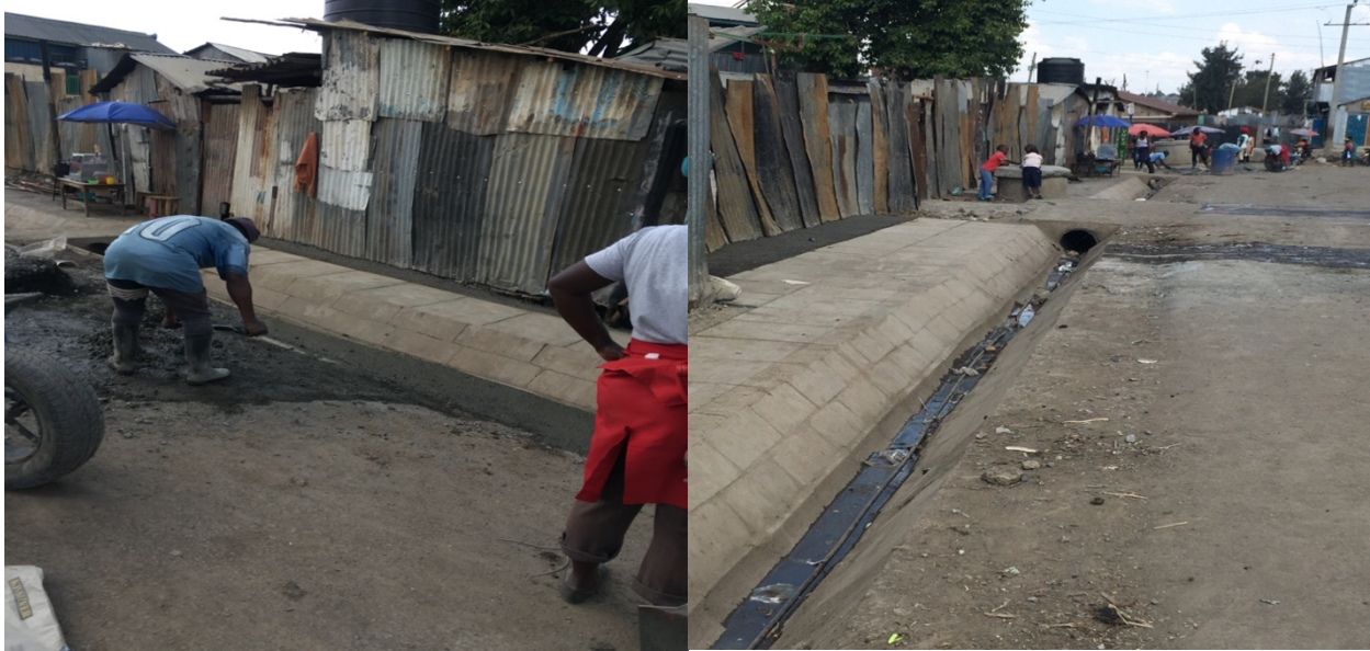
Fig 18: Ongoing road and drainage works in Kwa Reuben (Source: Author)
