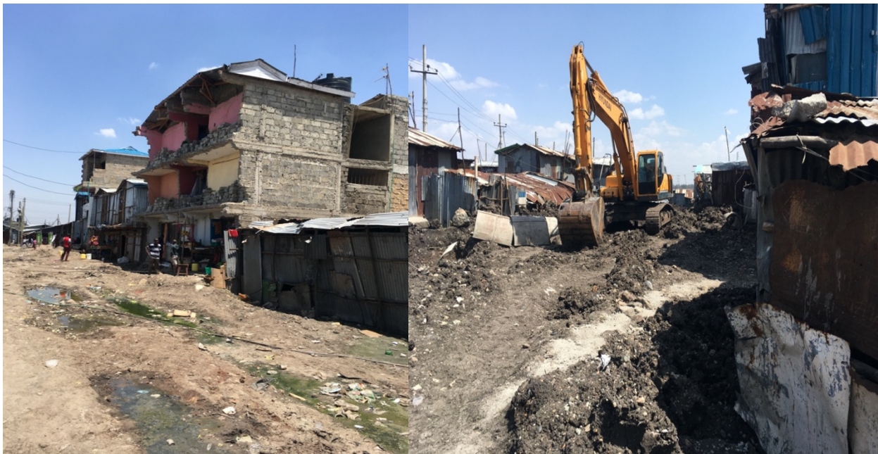
Fig 13: Demolitions carried out in Kwa Reuben and Viwandani (Source: Author)
