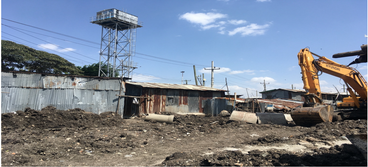
Fig 21: An elevated water tank at a borehole drilled with the onset of the COVID-19 pandemic, a sewer line is also being constructed in the foreground (Source: Author)
