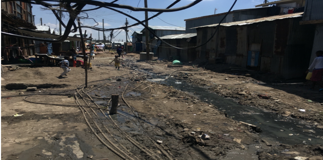
Fig 3: A section of a road in Mukuru kwa Reuben with unlicensed 'spaghetti water connections' running through (Source: Author)
