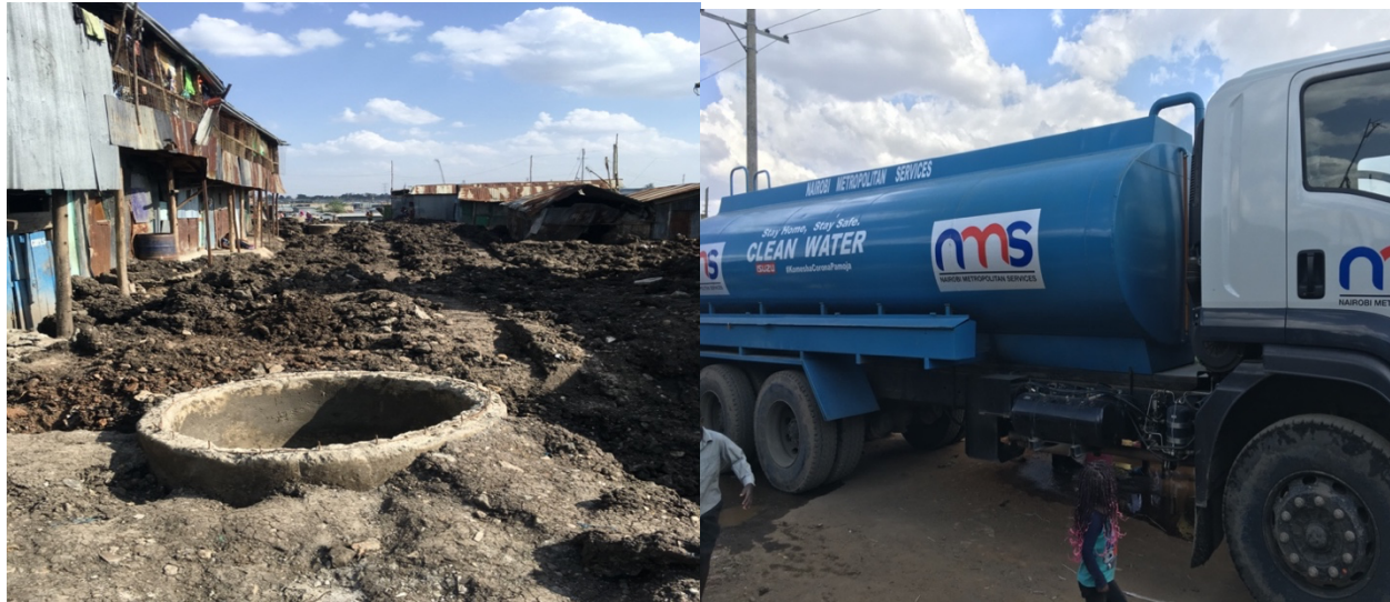
Fig 14: An open sewer pit recently constructed in Viwandani and a NMS truck supplying water in Kwa Reuben (Source: Author)
