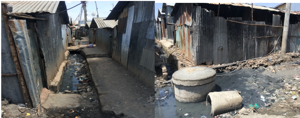
Fig 4: State of drainage in Mukuru (Source: Author)
